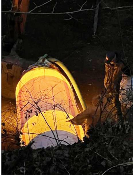
*Cured with safety sleeve to extend pipe to the desired length*
