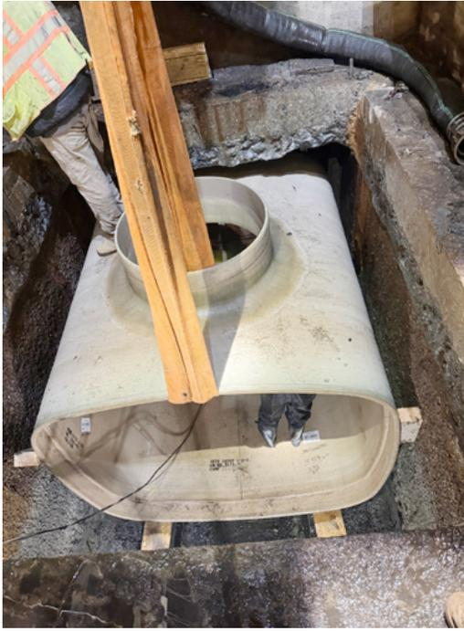
First Liner pipe with access MH for winch
