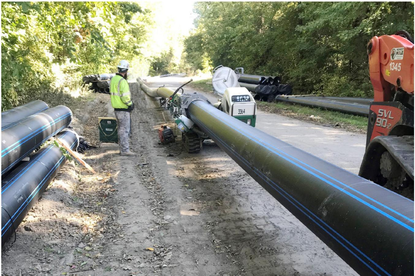
Nearly 3,000 feet of HDPE pipe for the under-the-river crossing was fused into one monolithic leak-free line
