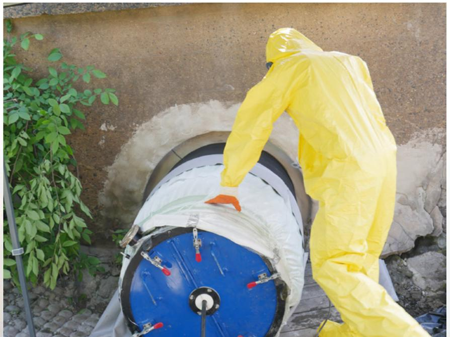
*The end gate (blue) had a port on the side for pressurizing with compressed air to inflate the liner. The cable attached was used to pull the liner into place*
