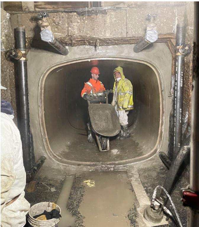
*High Side Bulkhead with 4-inch Grout Ports*
