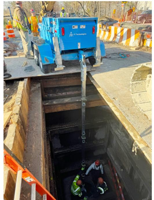
TT Technologies 12-ton Constant Tension Winch at Pull Pit
