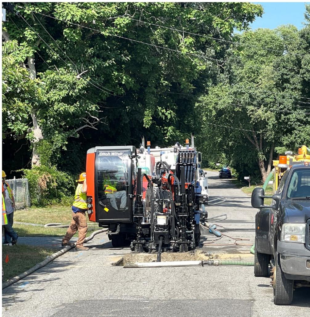
*Smaller and mobile HDD footprint was key to the efficiency of the installation*
