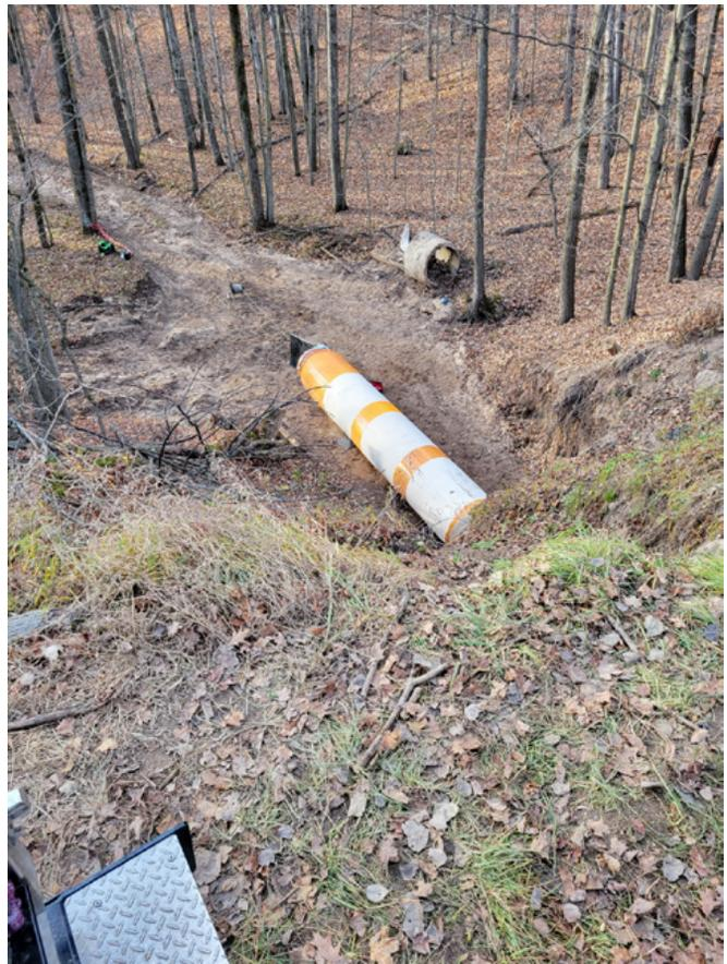
*Pipe was extended by 30 feet because the original pipe broke away and the road had washed out*
