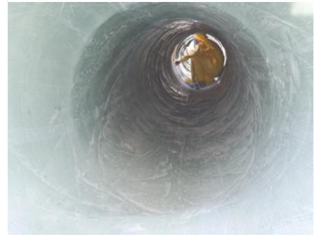
Using confined space entry, the final cured liner was entered to re-instate the center manhole lateral connection
