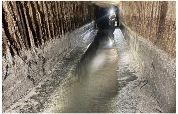
Existing 8 x 7-foot 1940s cast-in-place Interceptor Sewer to be HOBAS Slip-Lined
