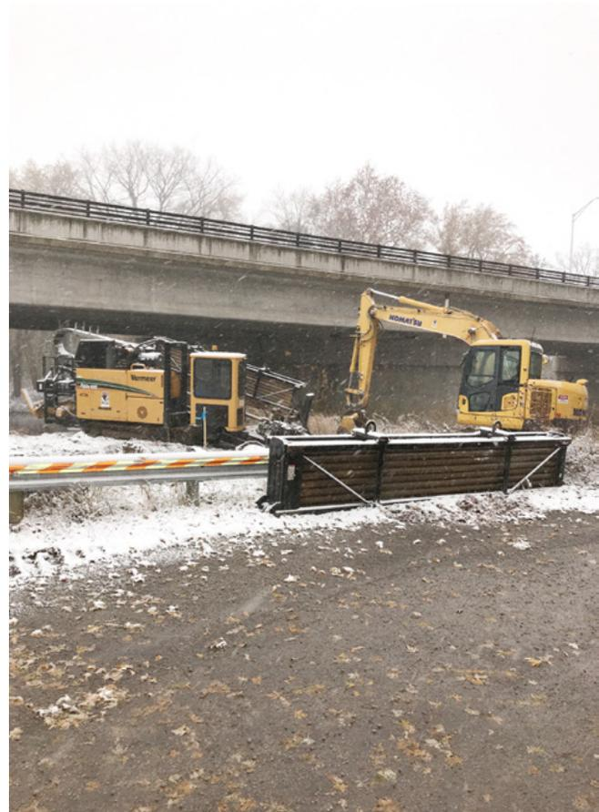
The HDPE pipe was installed 10 to 30 feet underground, parallel to the bridge on Maplecrest Road
