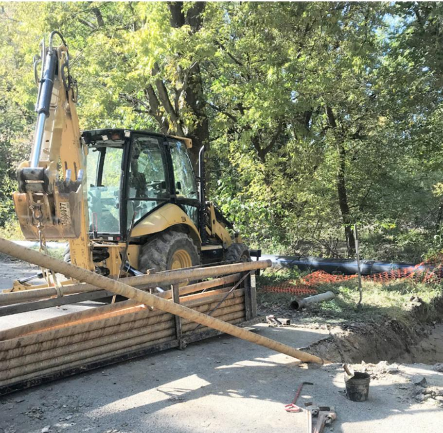
The Midwest Mole three-man crew used a fluted reamer with a cutting rig which was able to bore a path through the clay and cobblestone
