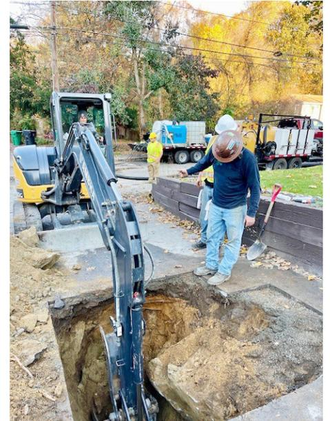
Geology was predominately hard pan with large cobbles and boulders, sitting on an outcrop of shale rock
