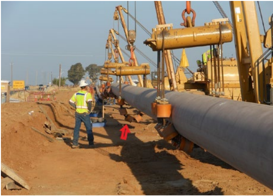
Having a safety factor of two for sling spacing can mitigate overstressing of the pipe during lifting into place by accounting for field conditions and human error
