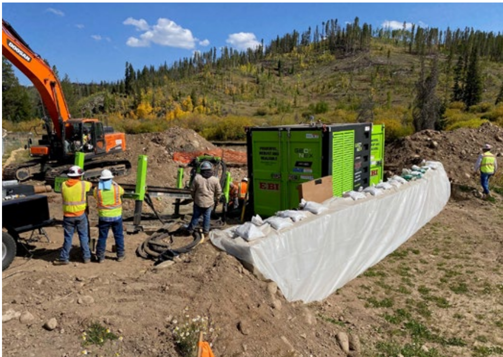
Drilling needed to go 240 feet through cobbles before hitting bedrock
