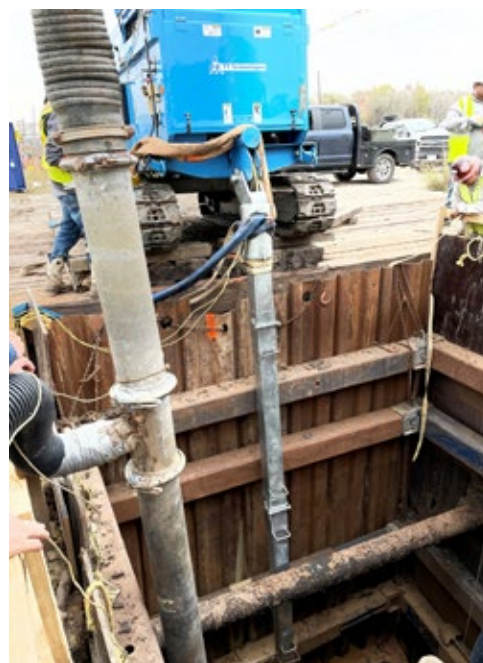
The variable speed Grundowinch makes adjustments for conditions that impact line speed during operation, providing constant and consistent pulling force
