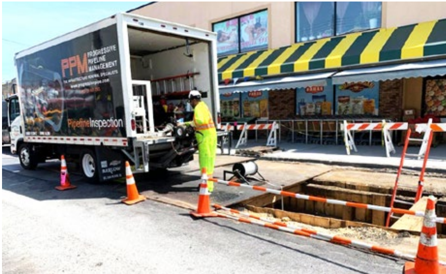
PPM crew with ARIES LETS CCTV camera used to inspect the pipeline prior to lining
