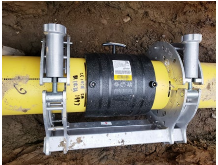
A properly prepared EF Coupling with Clamp
