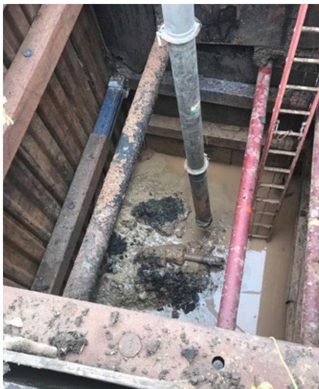
Soil conditions and a high water table meant crews needed to keep the dewatering pump in the pit running constantly to handle the ground water
