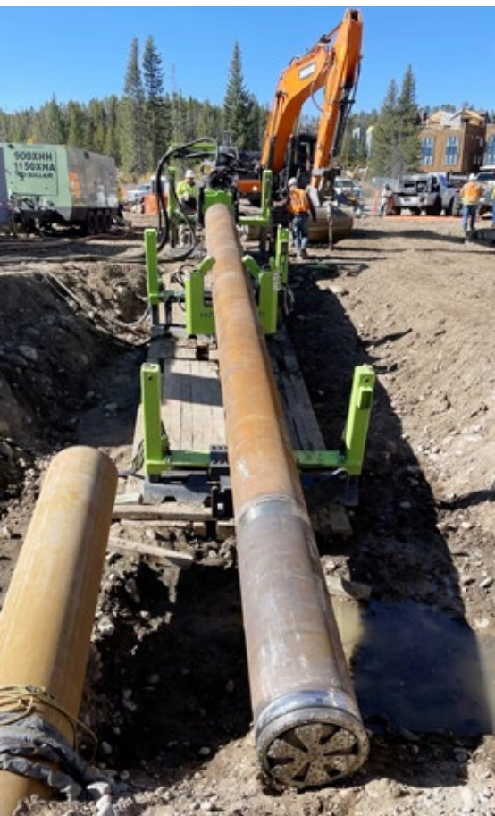
Down the Hole (DTH) Horizontal Hammer Boring was selected as the best method to install the 300 feet of 24-inch conductor casing
