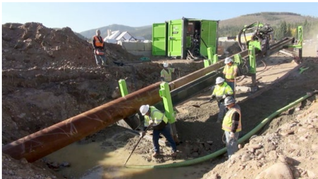
Geonex allowed the contractor to install the conductor casing twice as long as traditional hammer boring methods
