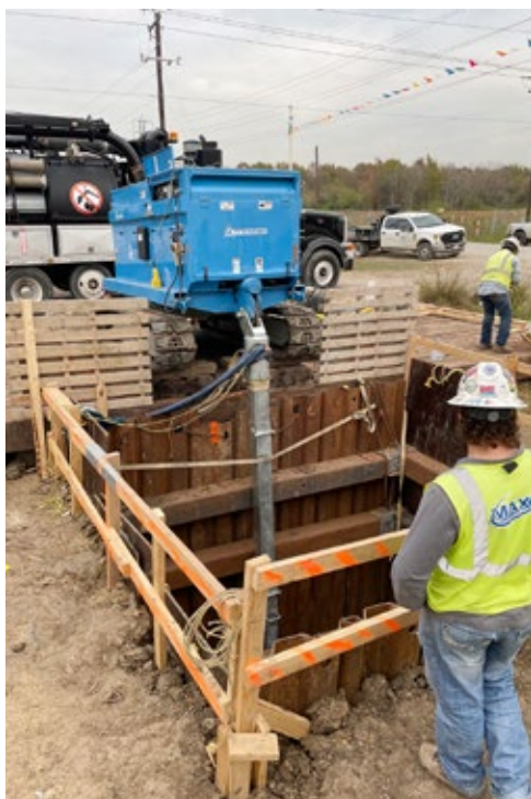
MAXX HDD crews drilled out to a 26-foot-deep pit, then used the winch to pull in the new pipe. The versatile “trenchless” winch provided the pulling power and the constant-tension needed to install the pipe without any issues
