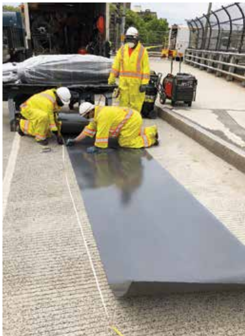
Preparing the Structural Reinforcement Sleeve (SRS) for installation in the bridge abutment
