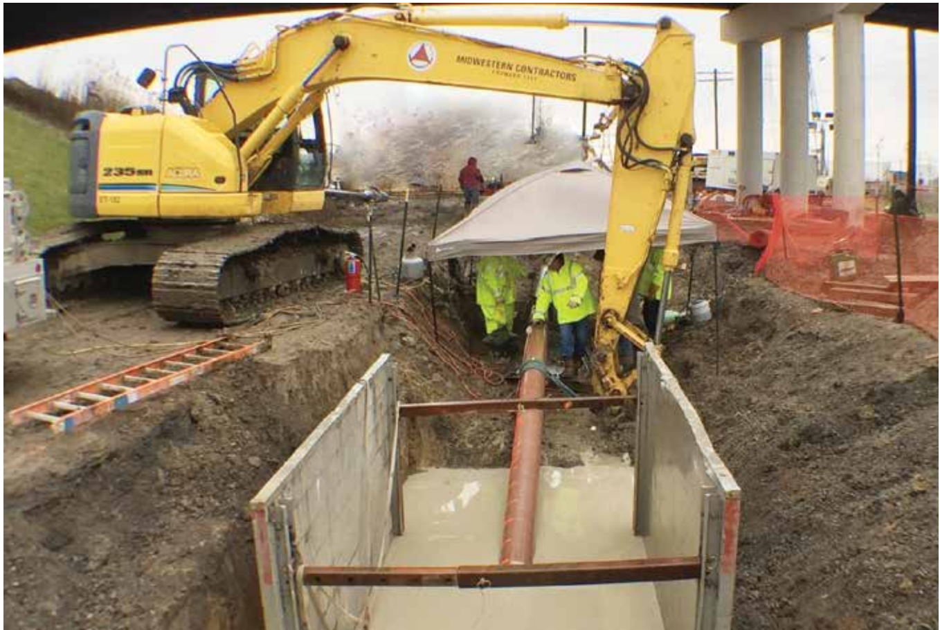
A containment pit for bentonite drilling mud to coat the pipe as it entered the ground was created on the push end of the project
