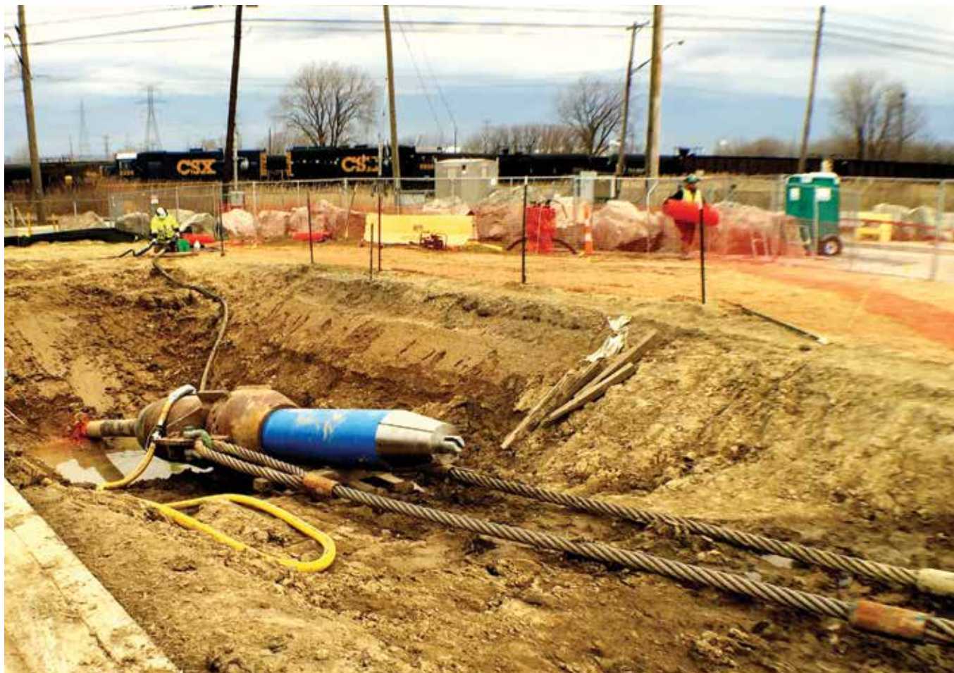
Midwestern Contractors extracted 2,400 feet of 12-inch steel pipe utilizing a combination of pneumatic pipe rammers and static pull force
