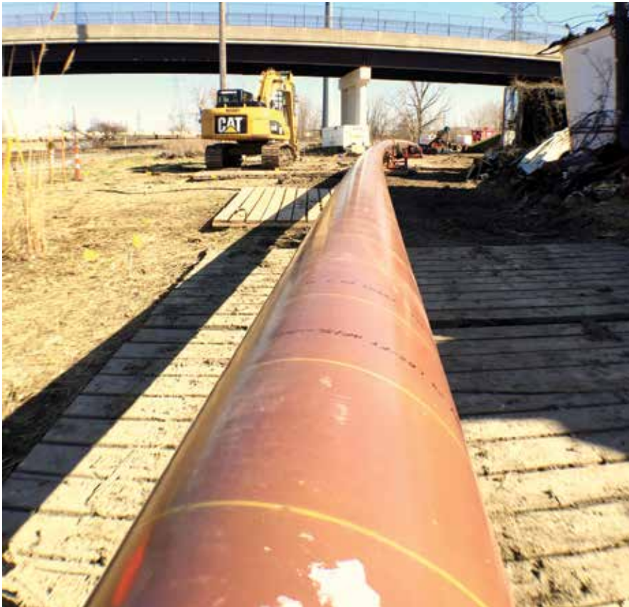
The contractor was able to extract the 2,400 feet of heavy wall pipe, weld and hydro-test a new pipe string and pulled it in behind the old pipe in four weeks
