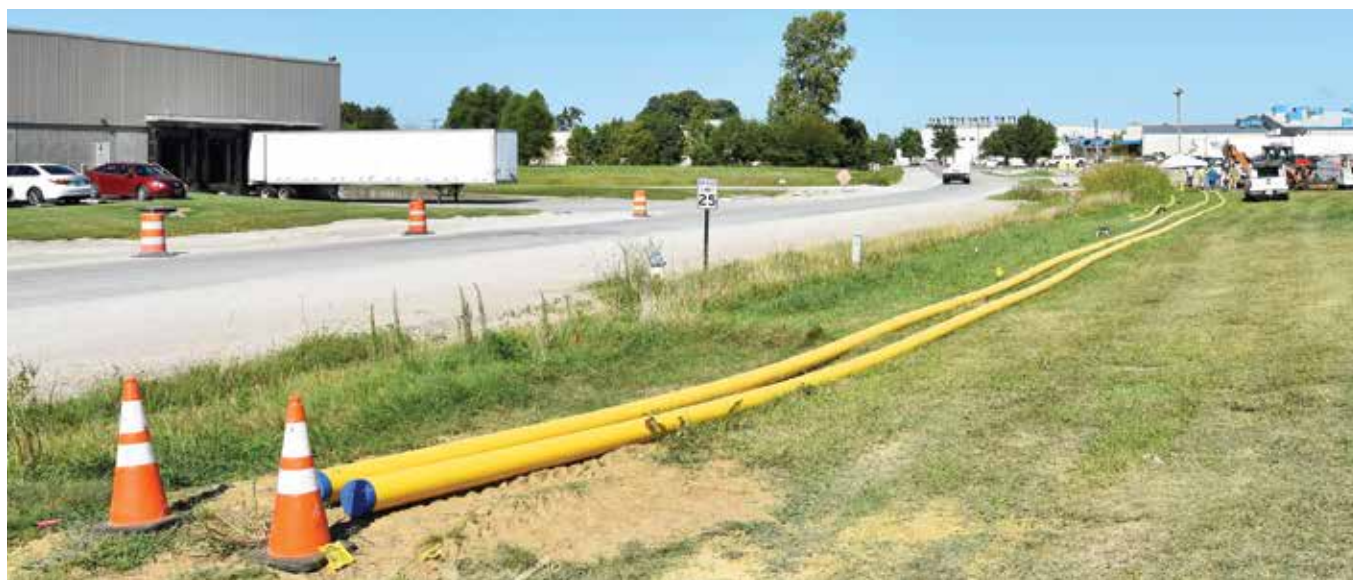
Two 750-foot-long sections of pipe were installed with HDD
