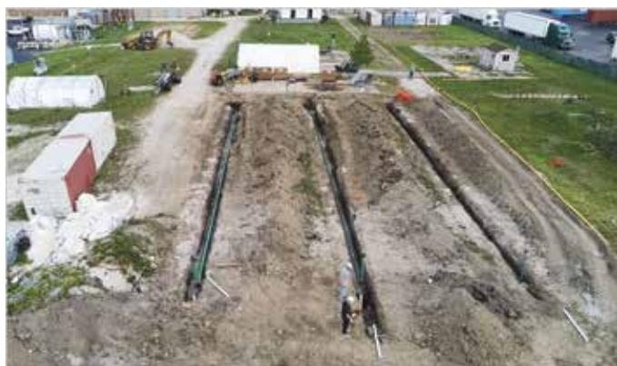
Figure 3. Aerial Image of Installed Pipe System from a Drone (Top of the Image is Facing East)
