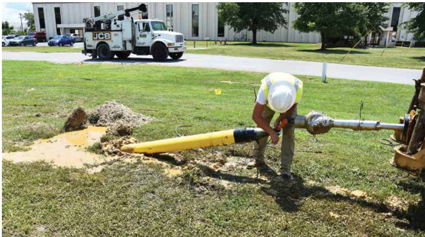
Installation went smoothly and none of the weak links or pipe were damaged
