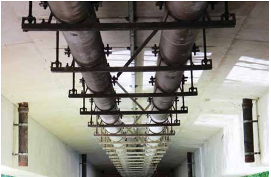
Bridge with pipeline hanging under bridge
