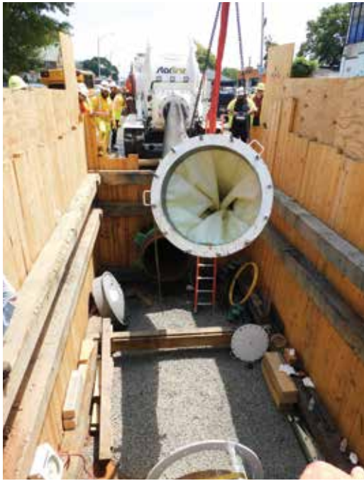
Readying a 42-inch gas main for liner inversion
