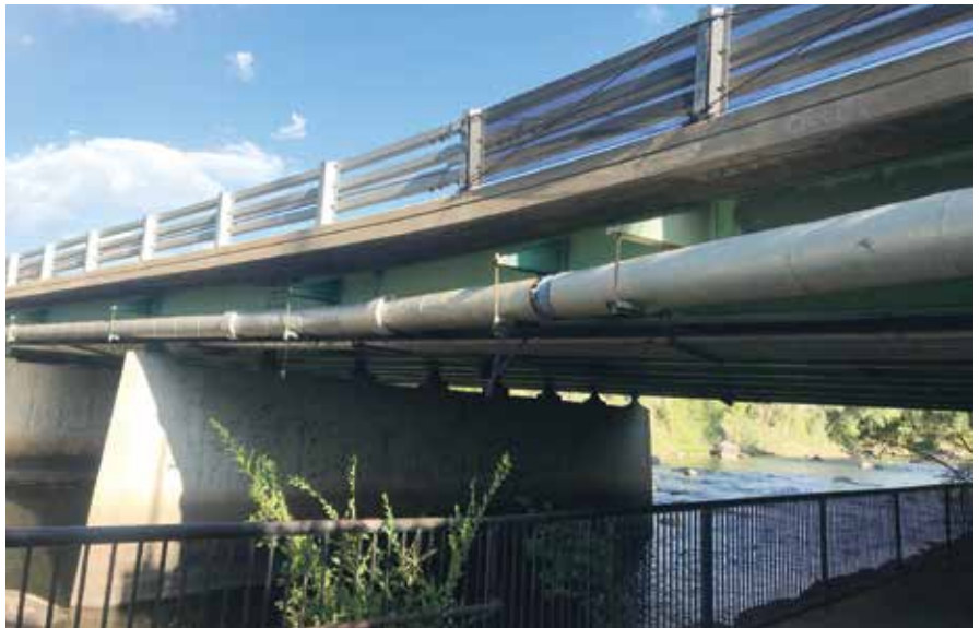
Bridge with pipeline alongside
