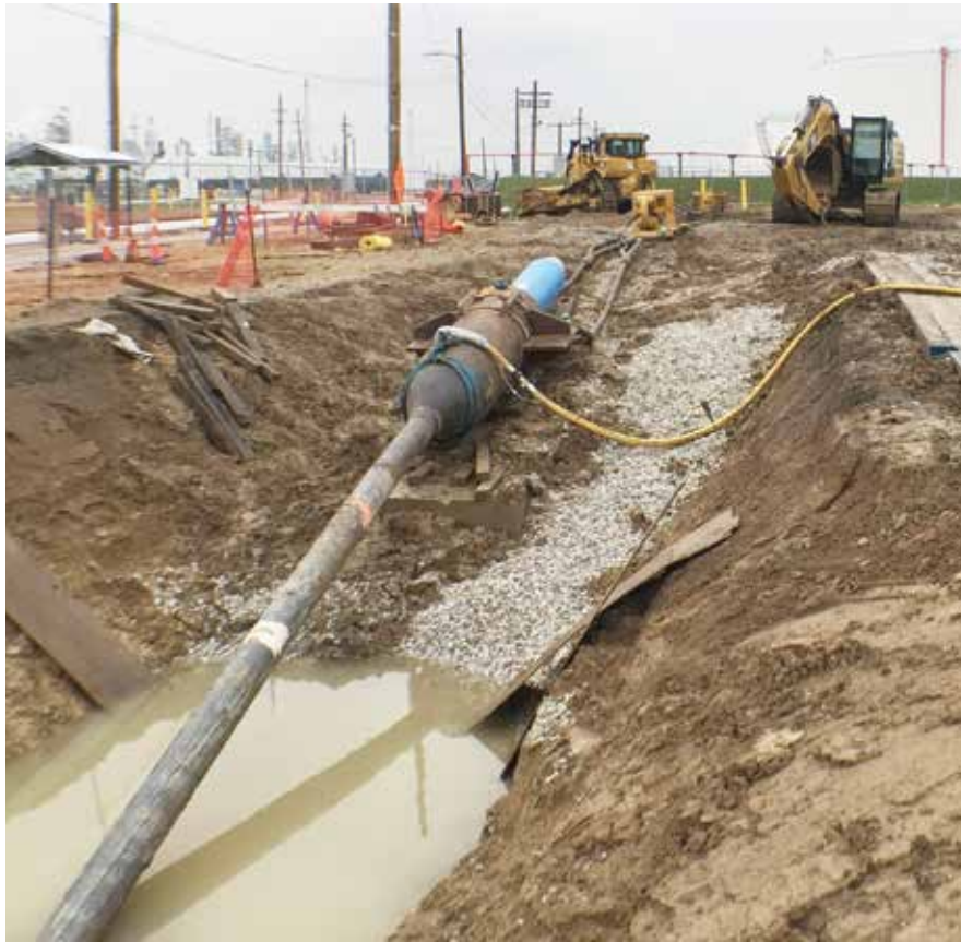
On the pull side of the project, the pneumatic rammer was used in conjunction two the D8 CATS and a 10:1 block system. Grundoram pipe rammers from TT Technologies were used for the percussive force
