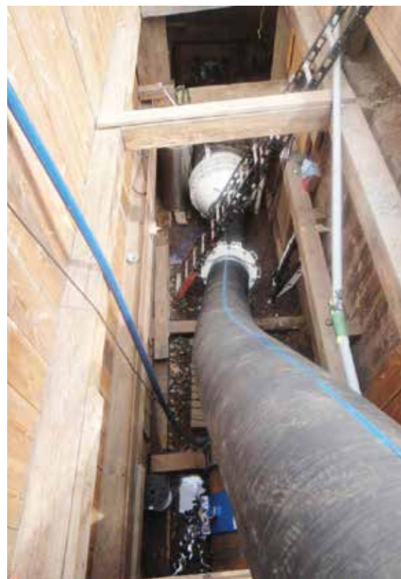
Transport hose used to convey inverting liner down into 10-foot deep pit. This innovation eliminates chafing during liner entry and is referenced as the “US Method”
