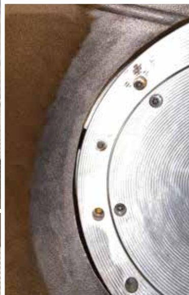
Design engineered prefabricated metal plug installed to cover a 20-inch lateral and provide bearing surface for liner inversion
