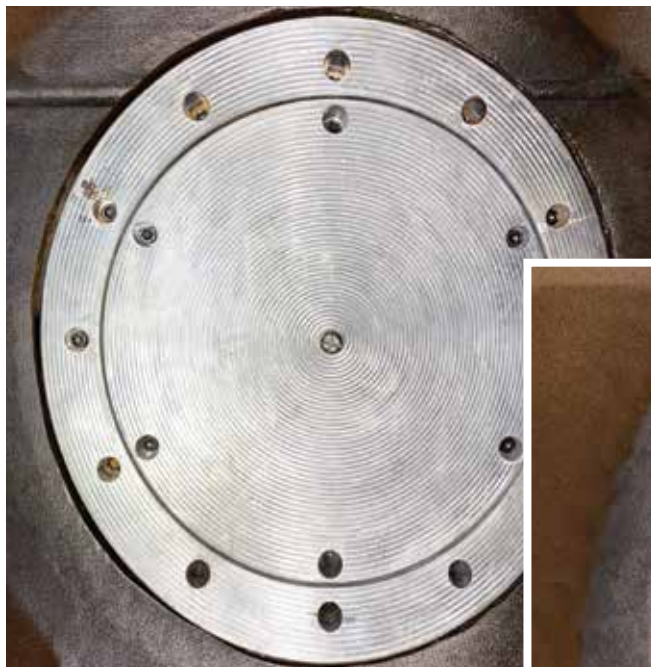
Design engineered prefabricated metal plug installed to cover a 20-inch lateral and provide bearing surface for liner inversion
