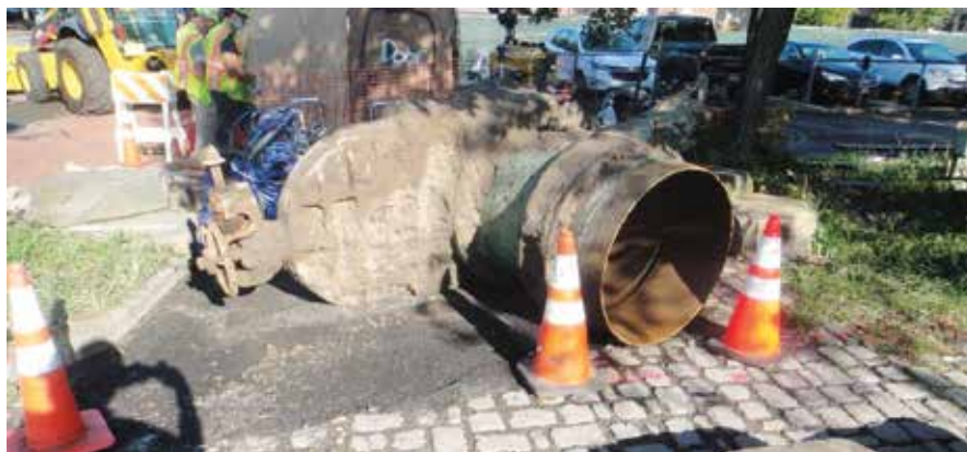
36-inch Valve was excavated on the east side of the “The Mess” to form the Receiving Pit for liner inversion
