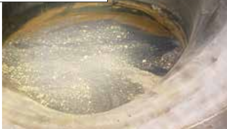
Stack was backfilled, then covered with mastic epoxy to form a 90-degree elbow from the 36x36-inch Tee
