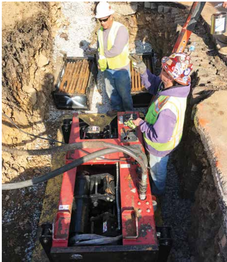
Hydraulic rod-pulling machines are typically used for steel pipe and larger plastic pipe slitting operations. This rod-pulling machine is being set up for a 460-foot-long, size-on-size replacement of 4-inch steel gas line with 4-inch MDPE.
