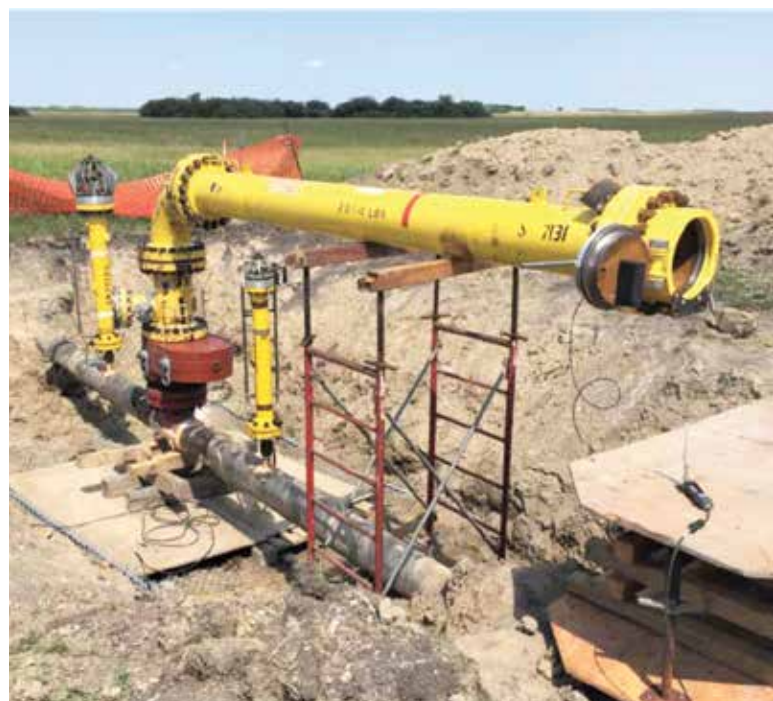
Figure 6: Pipetel's Launch System for Explorer 10/14
