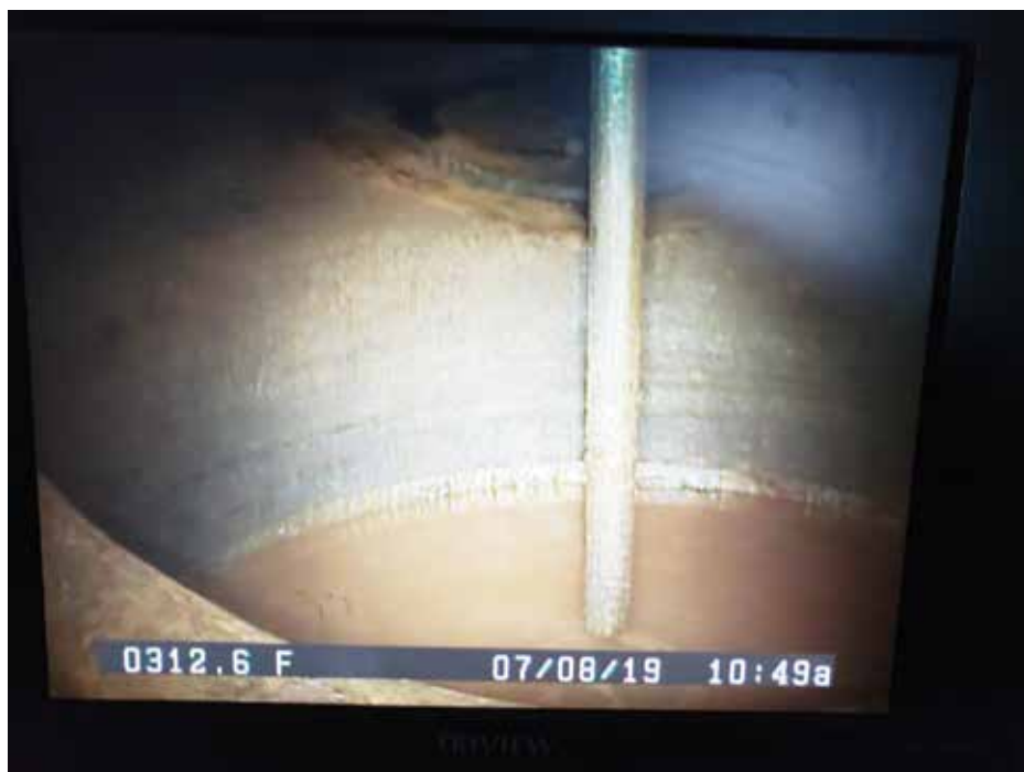
More than 70 gallons of water collected in the drip pot a week after main abandoned
