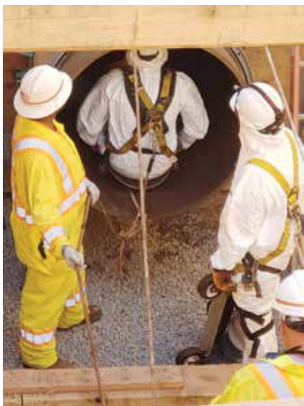
First-ever application of curtain grouting from inside a gas main required man-entry
