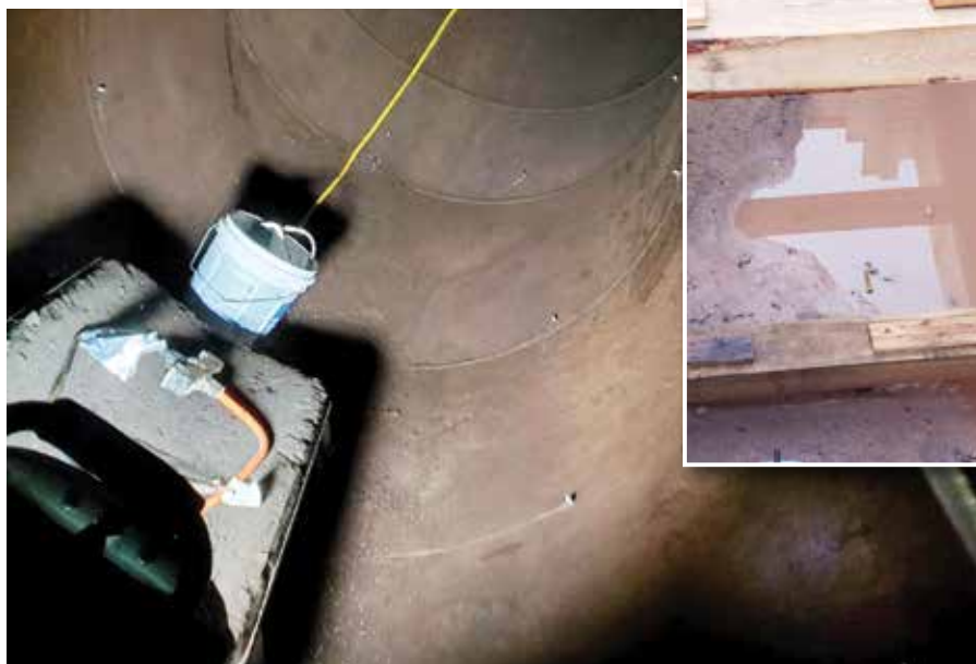
Grout pumped into soil through check valves stopped inflow from heavy rainfall
