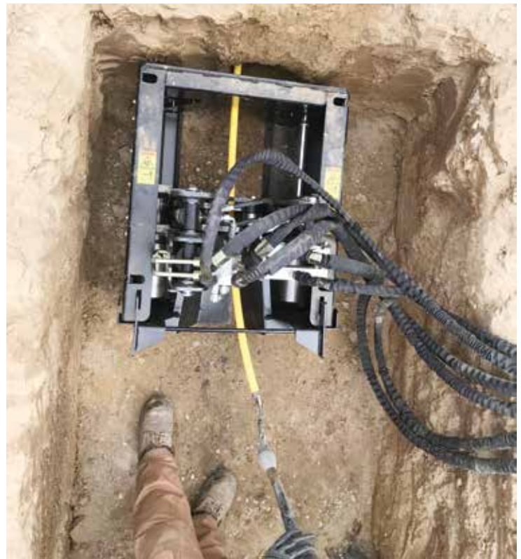
PE product pipe is pulled into place simultaneously as the existing pipe is extracted
