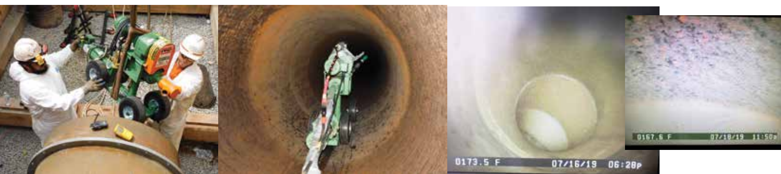
Self-propelled robotic sand blast unit, “The Beast” efficiently cleaned the metal to a NACE-2 finish
