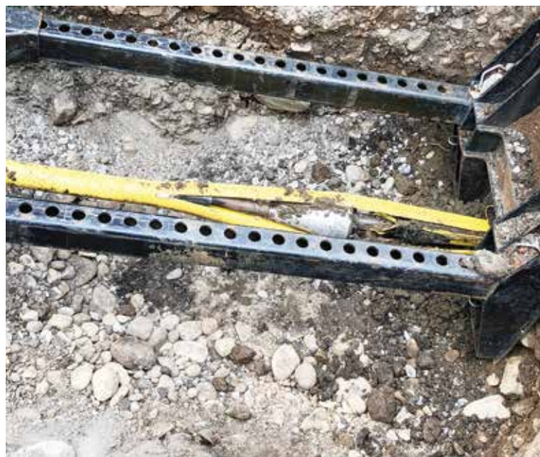
Trenchless pipe slitting is a proven method for replacement of plastic pipes that utilizes the same location as the existing line
