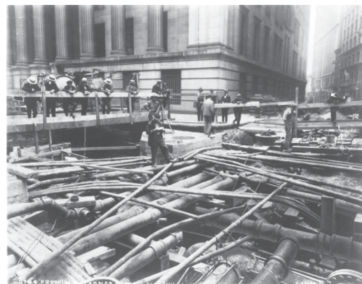
Example of ground congestion at the corner of Wall Street and William Street, Manhattan 1917
