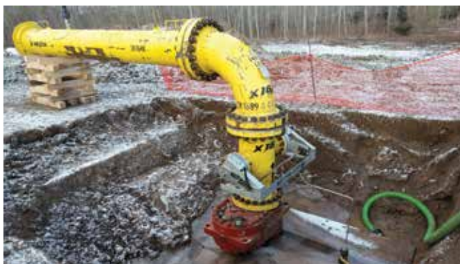
Figure 4. Sandwich valve isolating pipeline from launch tube used for Explorer to enter and exit pipe
