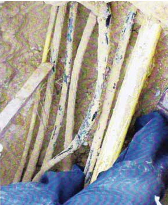
Multiple utilities are safely exposed in a common trench (gas, electric, and fiber). Probe shows hole where high voltage electric line faulted.
