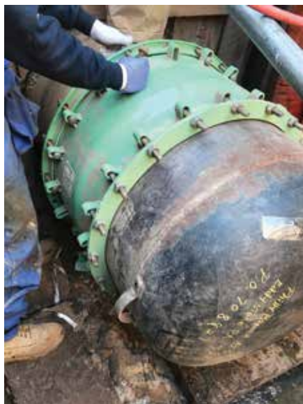
End cap bolted to pipe at end of day. Utility crews moved road plates, and removed end caps each morning
