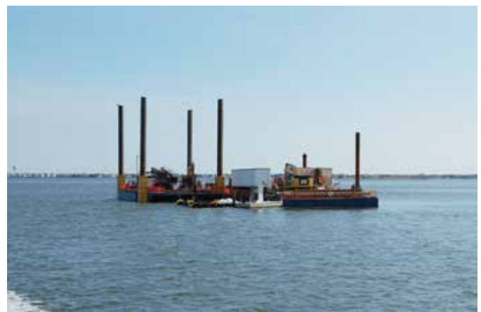
Figure 10 - Long Beach Island, cofferdam site
