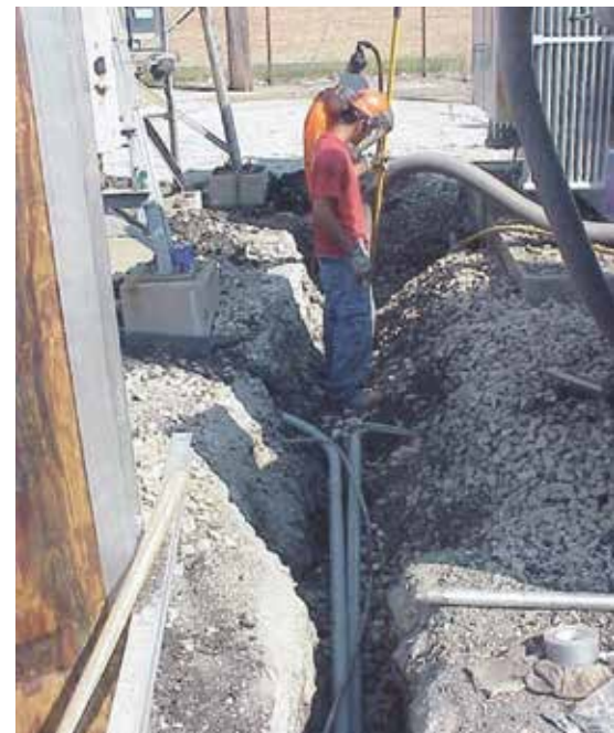
Vacuum excavating over buried control lines INSIDE a high voltage power station
