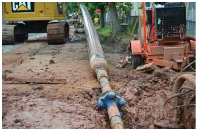
Start of pullback operation
