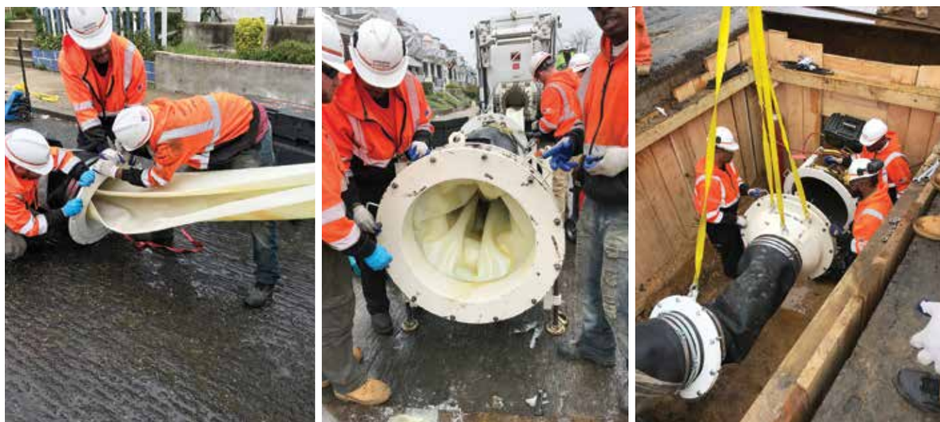
Liner is readied for installation. An incredible length and volume of 30-inch liner is being used – a combined total length of 3 miles of CIPL pipeline rehabilitation
