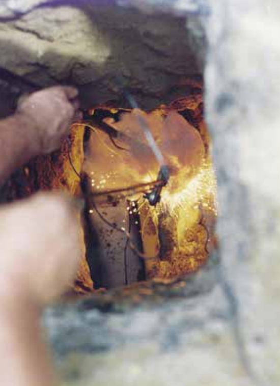
Attaching anode for cathodic protection to steel gas line using cad welding
