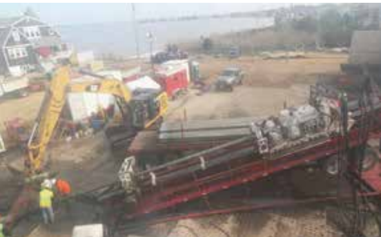
Figure 11 - South Seaside, HDD pull site, Seaside Park
