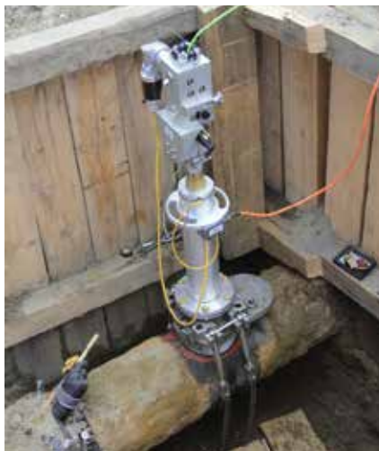
Small VGC Launch Tube installed on a 16-inch cast iron gas main for CISBOT pre-inspection
