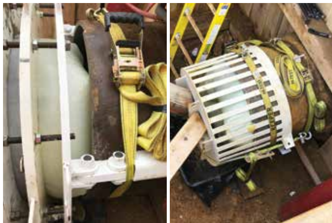
Liner is inverted through host pipe with continuous air pressure until it reaches end catch. Some lining segments are over 800 feet
