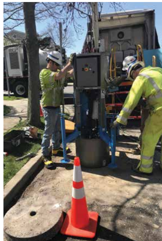
Grundopit K Keyhole Drill from TT Technologies was developed to bridge the gap between keyhole work and pipe installation. The mini directional drill is able to work within a 24-inch diameter core.
