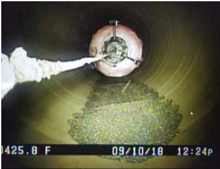
Custom pig was fabricated to remove stranded grit by reducing annular space to increase air flow
