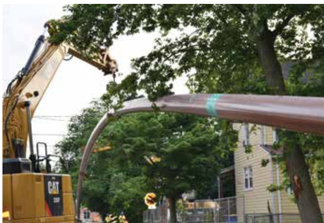
Maneuvering the last string of 16-inch pipe
