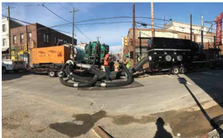
Optimal vacuum setup for cleaning 30 & 36-inch CI pipe before lining is equivalent of 7 separate vac units
