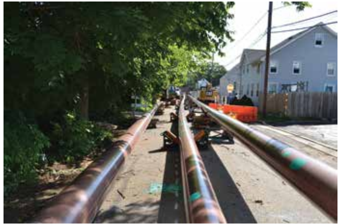
Three 400 foot strings of 16-inch pipe were staged on the exit side of the river
