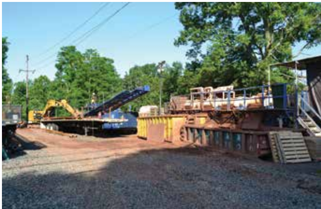
Drill, Bentonite Mixing & Recycling Rigs
