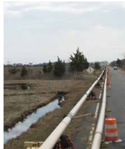
Figure 5 - South Seaside, pipe strings awaiting pullback. The drill site is near the building in the distance
