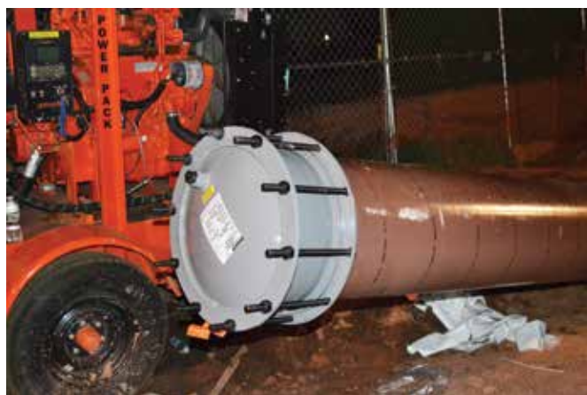
Pullback completion within 12 hours
