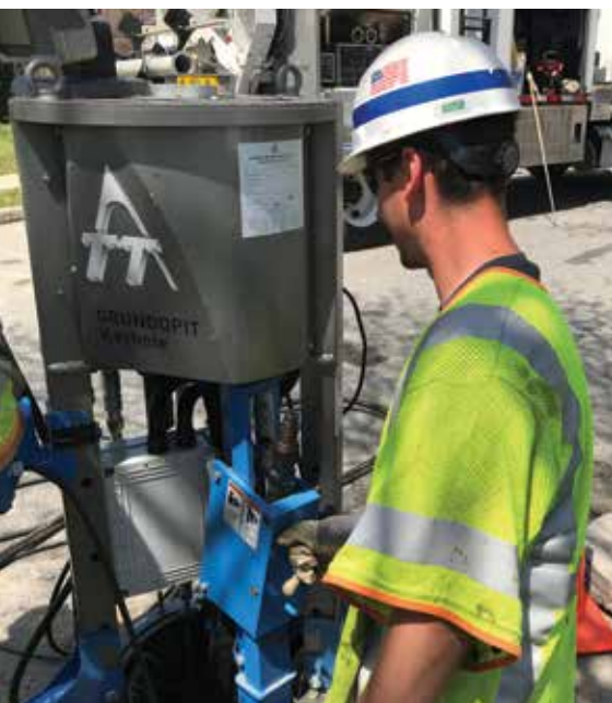
National Grid crews are able to control all of the keyhole drill's functionality through an above ground control panel.
