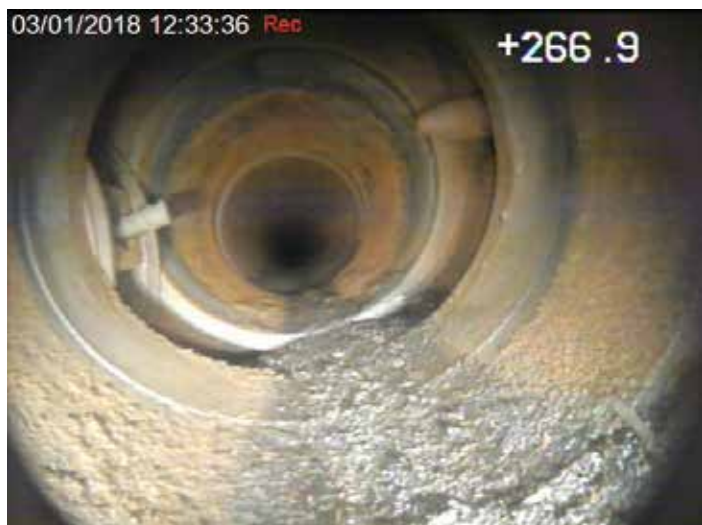
Gas main valve in open position
