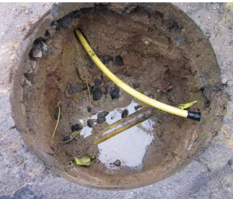
National Grid typically installs 1-inch MDPE services with the keyhole drill, however, the unit is able to install pipe up to 2 inches in diameter.
