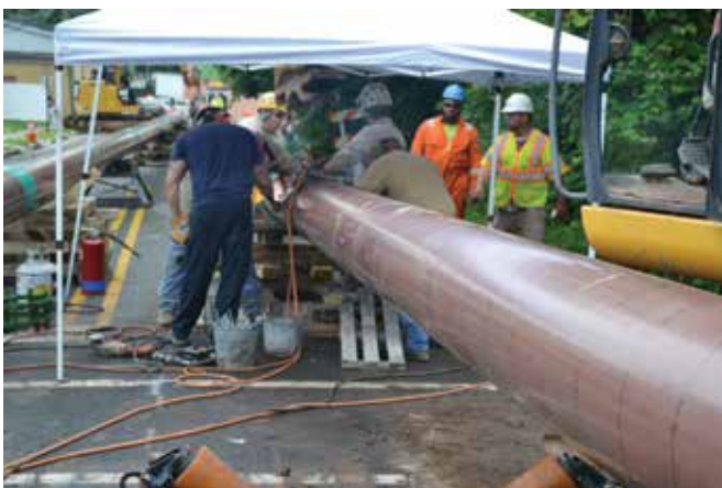
Welding of second string of 16-inch pipe
