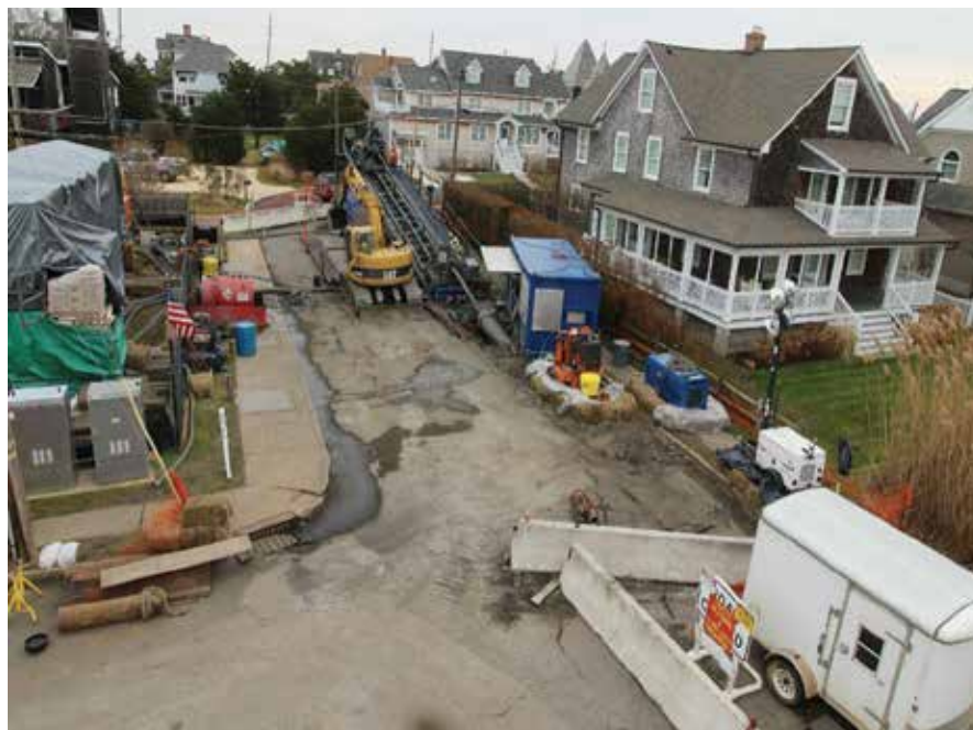
Figure 4 - North Seaside, HDD sending site, Mantoloking
