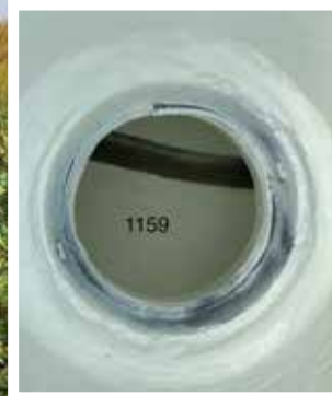
To finish the monolithic system and make it resistant to I&I, all 12 manholes were spray coated with 350mm epoxy spray using the same low toxicity aquatic safe epoxy that was used for the liner. Curing of the epoxy was assisted using a heater mounted at the top of the manhole. The complete CIPP system guaranteed the protection of the local ecology, with the pipe completely submerged in the ocean. The Town has acquired valuable experience in using epoxy CIPP to re-establish a pipe's structural integrity when situated below a tidally fluctuating water table.
