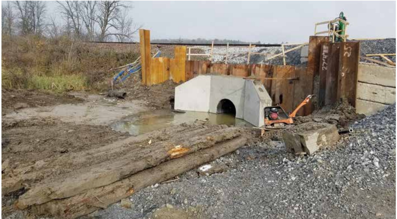
Culvert set-up during construction
