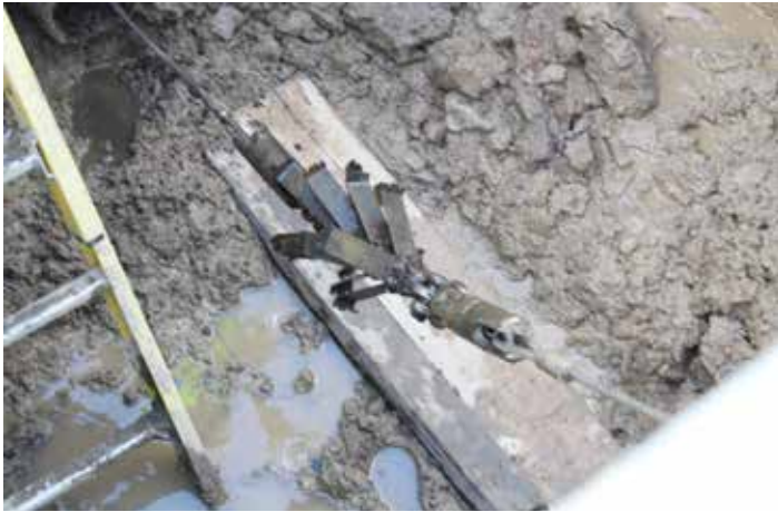
Pipe cleaned by drag scraping
