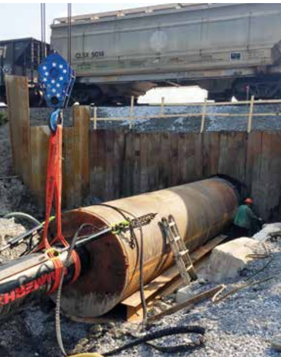
The pipe-ramming technique permitted rail service to continue unimpeded throughout the 6-month duration of the project
