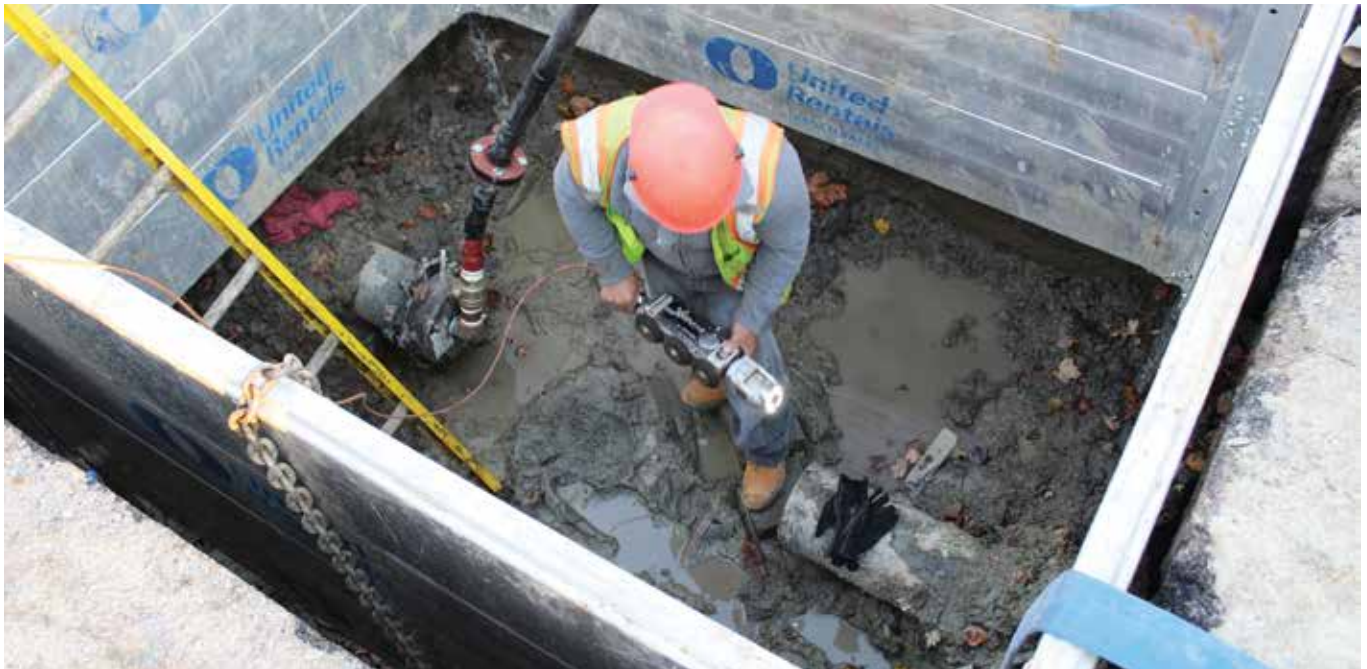
Camera inspection before lining
