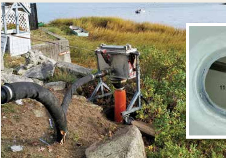
Rollers and mud mats were used to protect sensitive beachfront environment during installation of the CIPP liner below Sea Street, threading between the narrowly-spaced beachfront homes. Vehicles and equipment were located in the roadway approximately 100 – 300 feet away from each manhole.
