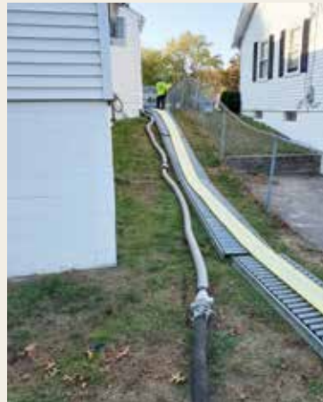
Rollers and mud mats were used to protect sensitive beachfront environment during installation of the CIPP liner below Sea Street, threading between the narrowly-spaced beachfront homes. Vehicles and equipment were located in the roadway approximately 100 – 300 feet away from each manhole.
