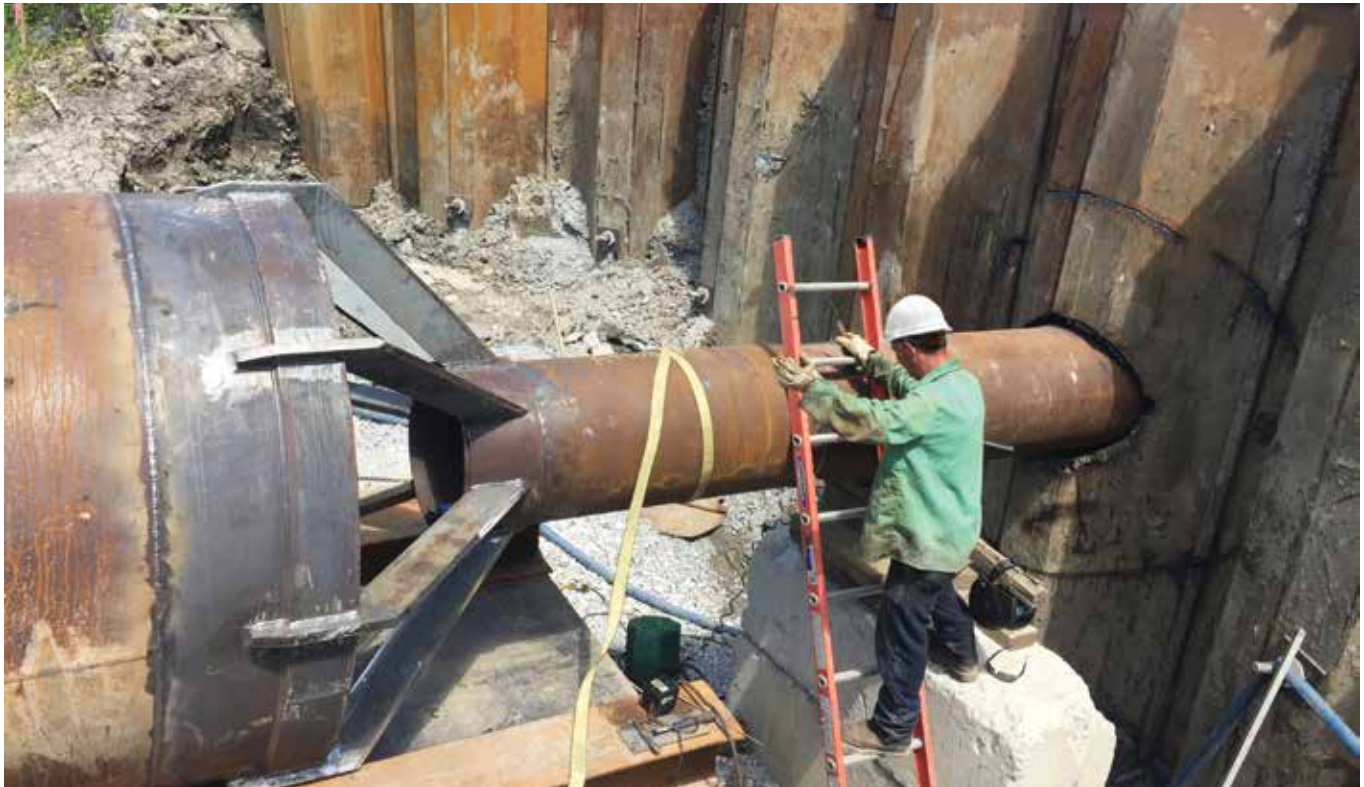
24-inch "Pilot Pipe" was used as a guide for ramming the 72-inch casing
