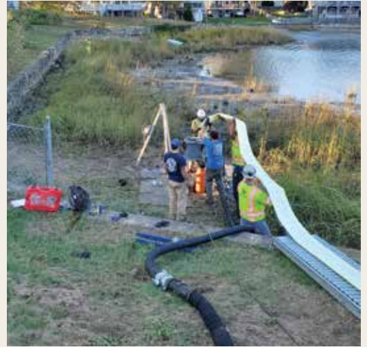
Tidal influence and high water table levels presented big challenges during construction. Installations were limited to a 6-hour low-tide window, lining approximately 300LF segments of pipe per day, in a tightly choreographed process.
