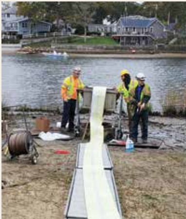
Rollers and mud mats were used to protect sensitive beachfront environment during installation of the CIPP liner below Sea Street, threading between the narrowly-spaced beachfront homes. Vehicles and equipment were located in the roadway approximately 100 – 300 feet away from each manhole.
