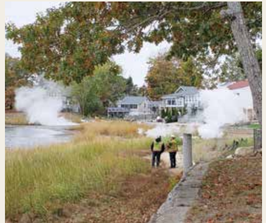
Due to the tidal influence bringing the liner into contact with colder seawater, steam curing times were increased to compensate. Curing time for most segments took nearly two hours.
