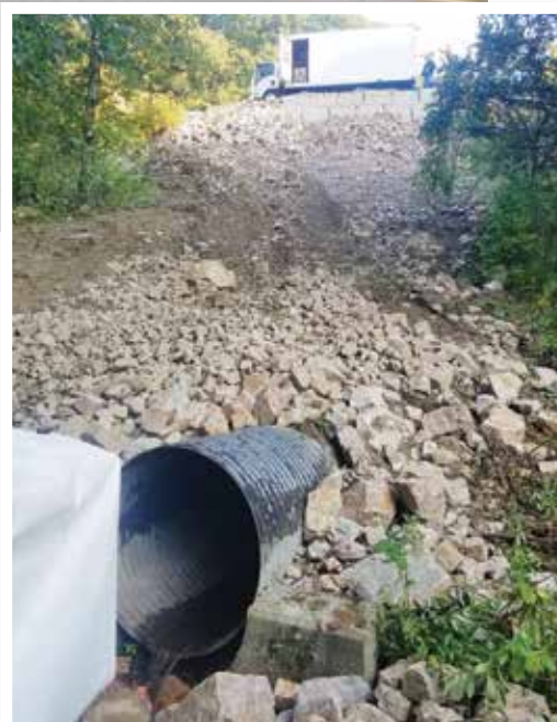
42-Inch Culvert looking up hill
