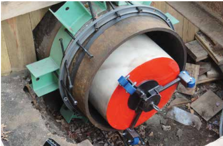
Custom pig fabricated to remove stranded grit
