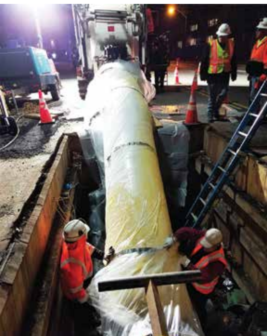
Starline® Cured in Place Liner coming off the drum guided as it enters the host pipe
