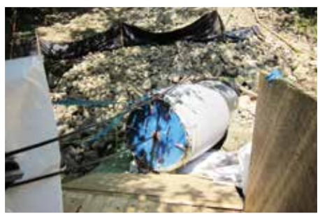
Liner installation took about 18 hours to complete
