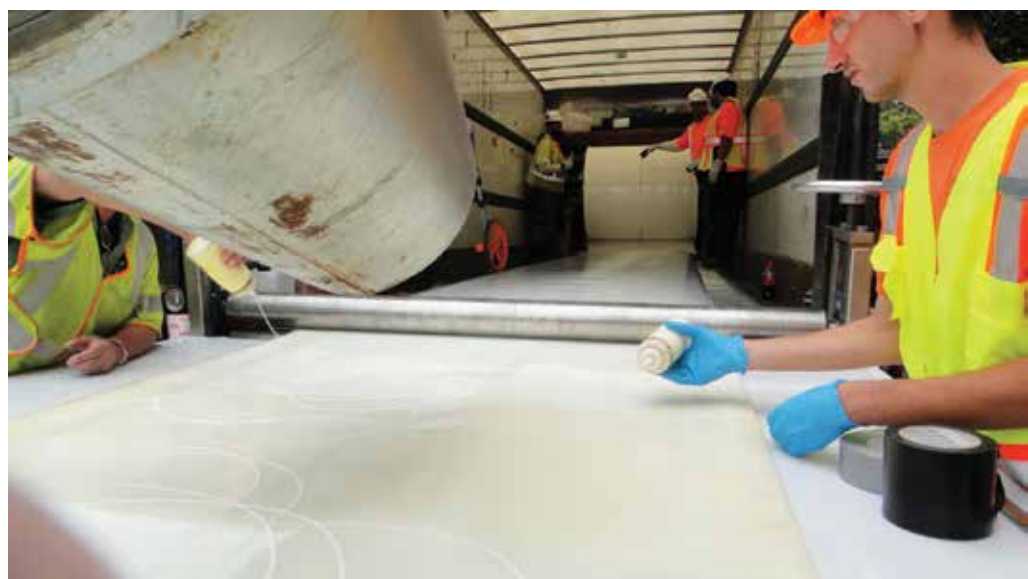
Liner wet out involves mixing two-part chemicals
