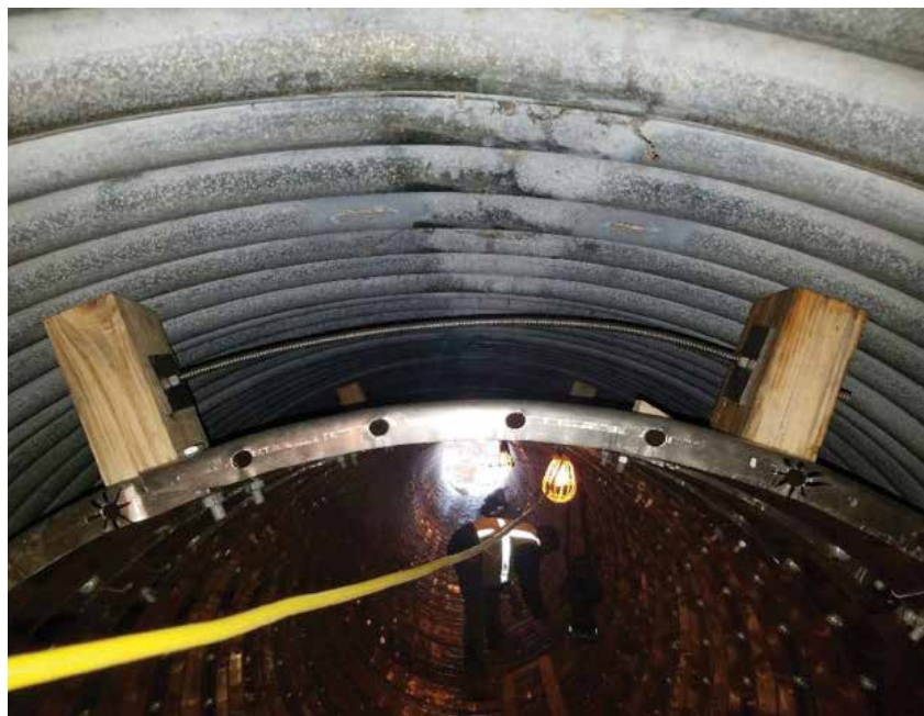
Blocking between Tunnel Liner Plate and host pipe ensured worker safety and provided uplift resistance during grouting
