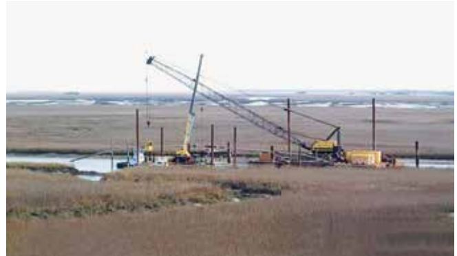
Figure 3 - HDD and cable splicing work platform within Hamlin Sound, SC situated in the marshland. The pipes carrying high voltage cables installed by HDD are being overboarded and buried below subsurface (Photograph courtesy of Pridmore and Varner/TD World.com)
