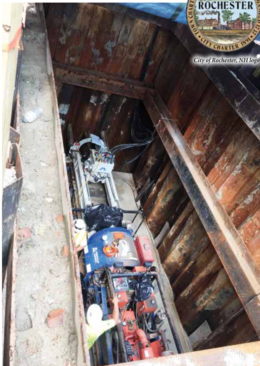
Steel Casing Installation by ECI using American Augers Boring Machine
