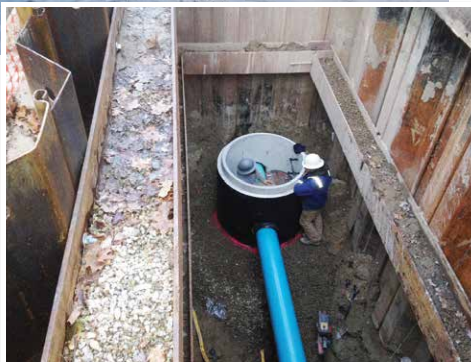
Termination of the Gravity Sewer Crossing into a Junction manhole
