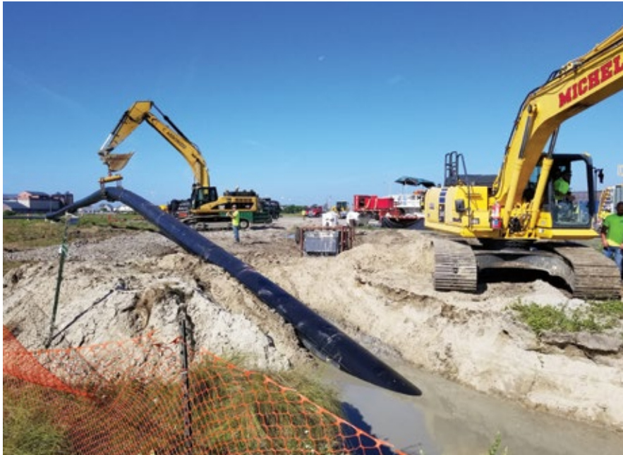
The 30-inch diameter HDPE PE 4710 pipe enters the HDD path to go under the Beach Thorofare waterway. (PHOTO COURTESY OF ACUA)
