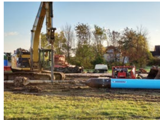
Figure 3. The 24-inch Fusible PVC® casing pipe ready to be pulled into the bore hole
