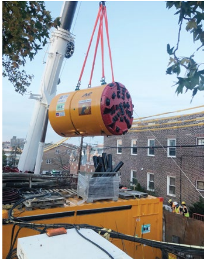
Figure 8: Lowering of MTBM AVN2000AB at Chamber 4 / Jacking Shaft
