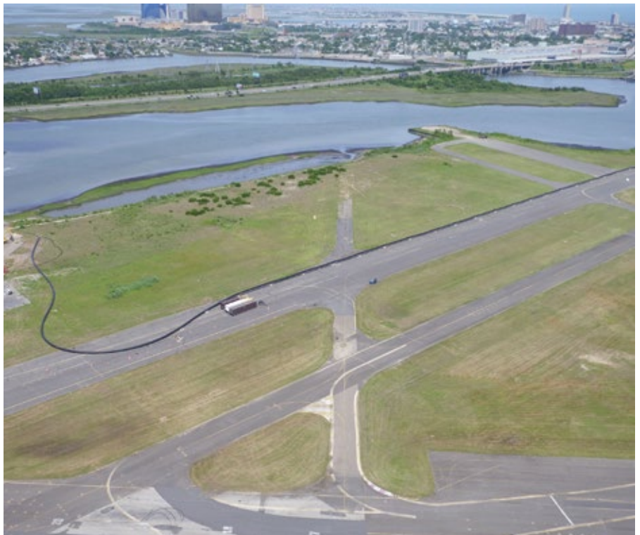
Heat fusing the sections of HDPE pipe was done and the resulting monolithic pipeline was staged along a runway at the former Bader airfield, ready for the 1,500-foot HDD pull 80 feet under the Beach Thorofare waterway. (PHOTO COURTESY OF ACUA)
