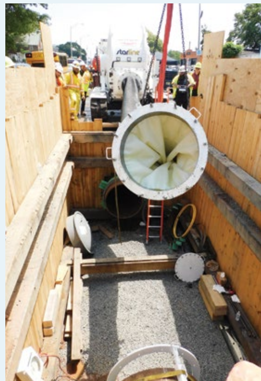
Leaking 42-inch cast iron gas main repaired using Starline® Cured-In-Place-Lining (CIPL)
