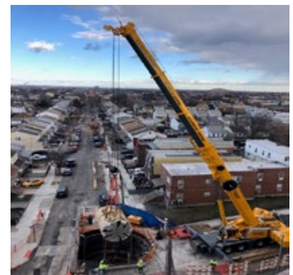
Figure 8: Lowering of MTBM AVN2000AB at Chamber 4 / Jacking Shaft
