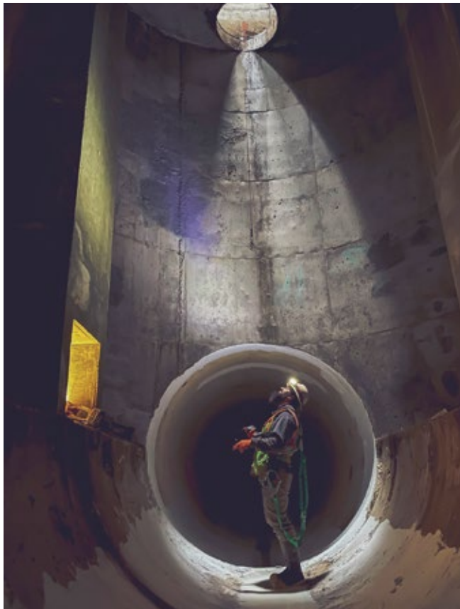
Figure 9: Final Walkthrough & Inspection of 96-inch RCP
