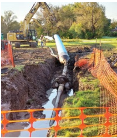
Figure 4. The 24-inch casing pipe being pulled into the bore hole
