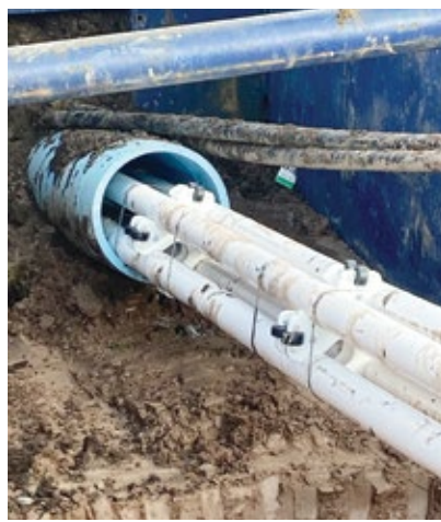
Figure 5. The 5-inch conduit bundle emerges from the bore hole
