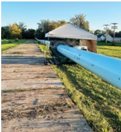
Figure 2. The fusion operation for the 24-inch Fusible PVC® casing pipe
