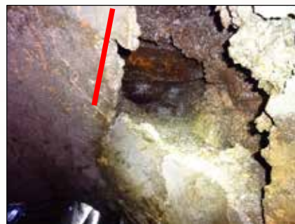
(d) Looking into void (downstream), approximately 10 feet deep.
