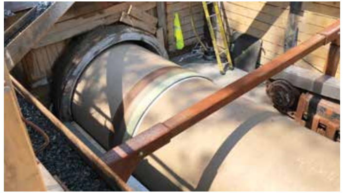
New pipe in-place
