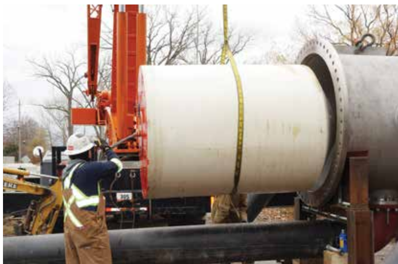
Figure 3.60-inch durafoam style pig being placed in launcher
