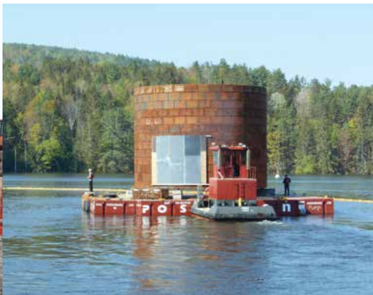
Figure 5: Water leg cofferdam structure with fiberglass soft eye
