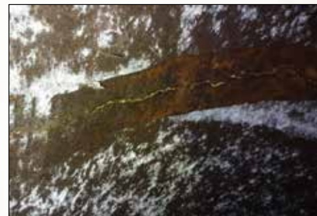
(b) Defect after dewatering.
