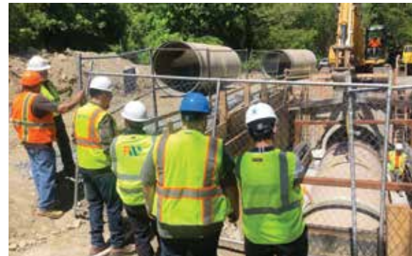
Field crew observing FRP slipliner getting pushed with one excavator and pipe pusher
