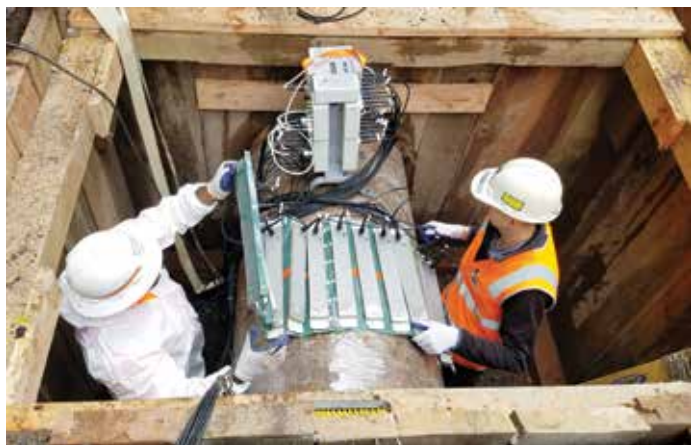
External NDT inspection of exposed CI pipe
