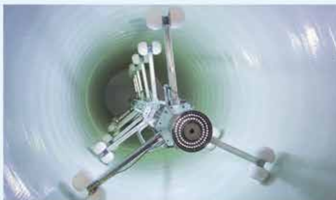
UV Mainline Lining
