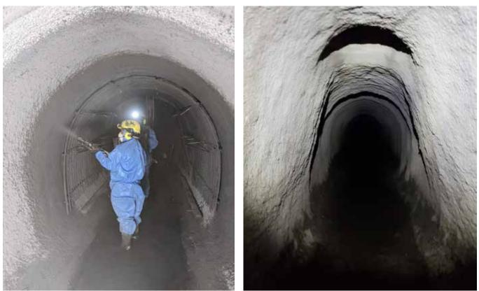
Spraying liner over basalt reinforcing bar (left) and completed manhole rehabilitation (right)
