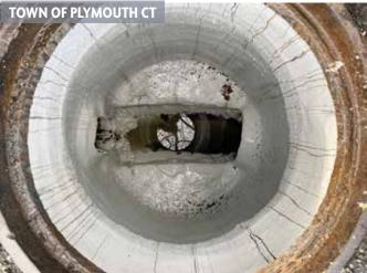
Figure 3. Completed rehabilitated manholes
