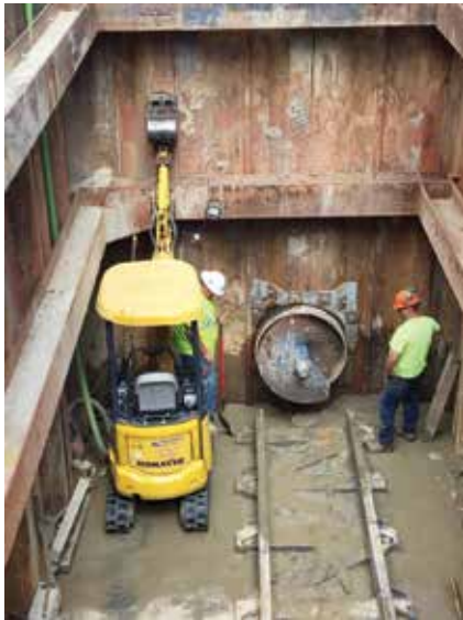
Auger bore through 42-inch casing
