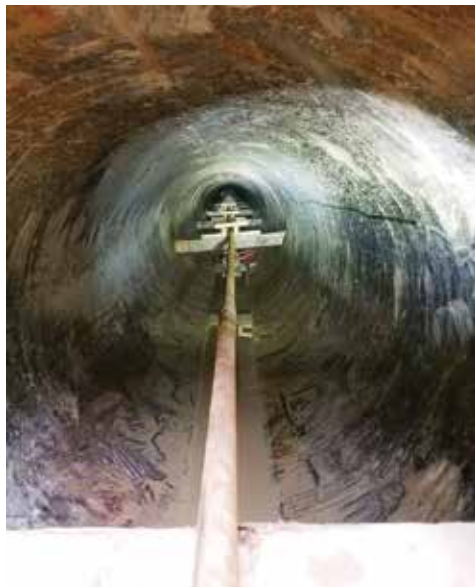
Pilot tube guidance system for the tunnel - Thinking out of the box.
