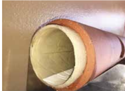
CIPP Liner Cured in Existing Pipe
