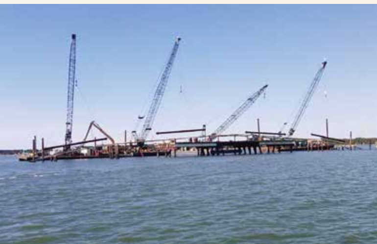
Overboarding pipe from fixed platforms for twin 17,000-foot HDD crossing of York River Power transmission project
