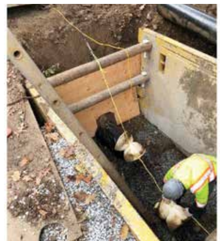
Squeezing the existing water main
