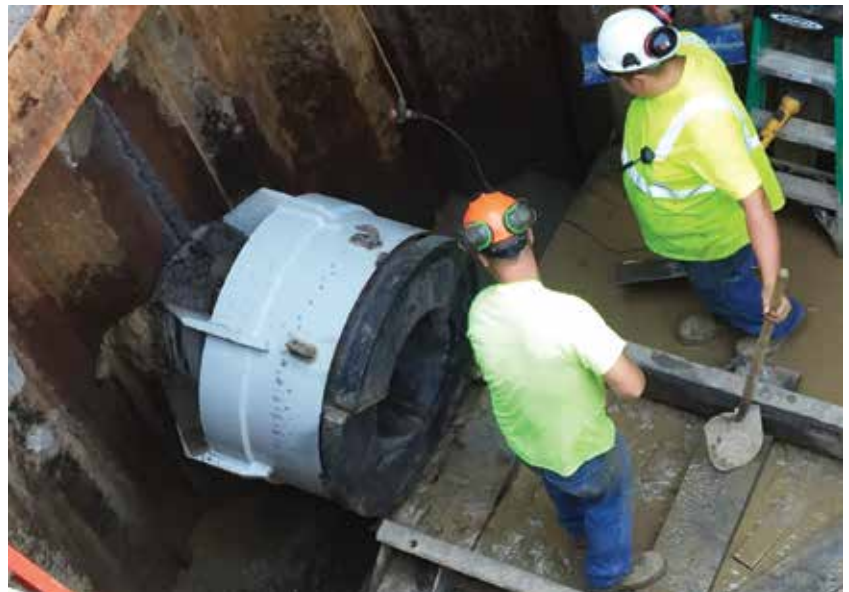
Akkerman weld-on reaming head
