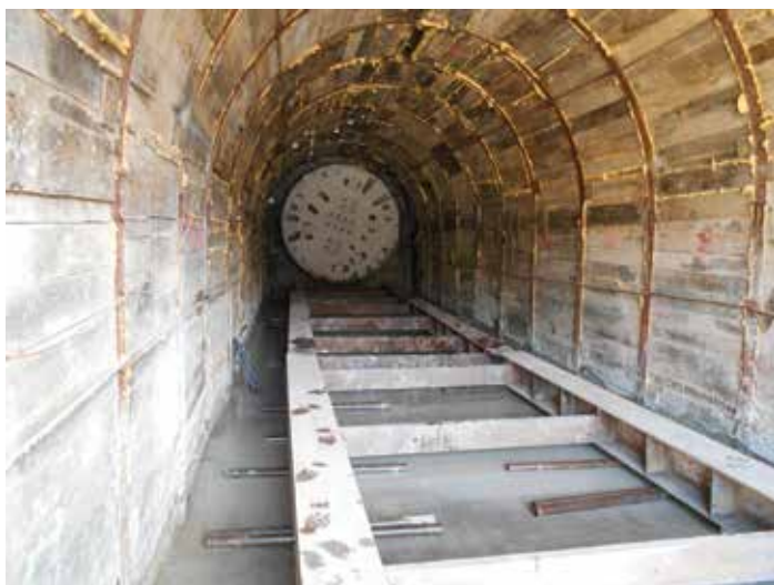
Figure 4: MTBM holed through into the hand-mined tunnel
