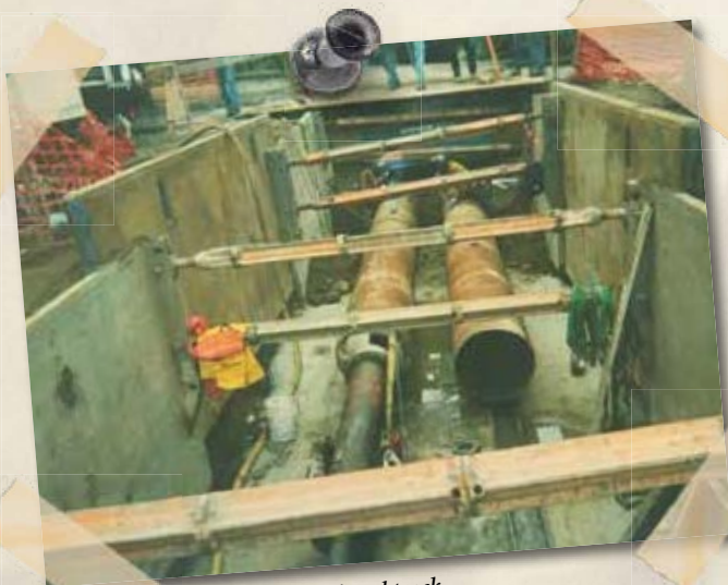
Two 30-inch casings under railroad track
