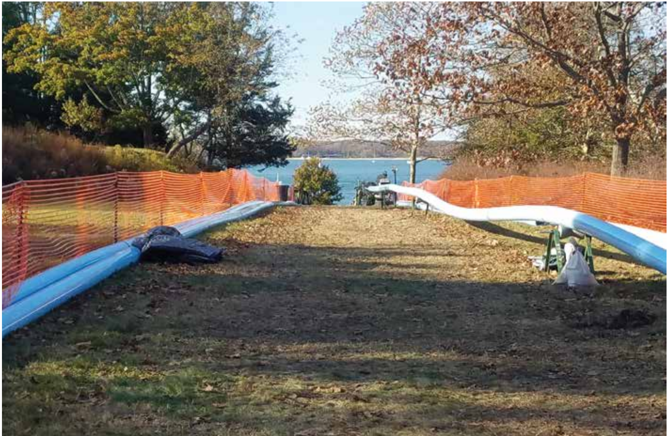
First of 3 conduits is pre-assembled for installation
