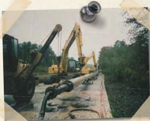
When directional drill is immobilized percussive power frees 2500 feet of 24-inch pipe with air hammer attached
