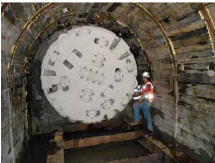
Figure 4: MTBM holed through into the hand-mined tunnel
