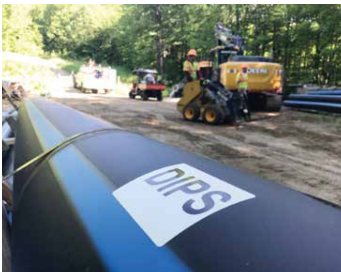
More than two miles of new 12-inch HDPE DIPS SDR11 pipe installed
