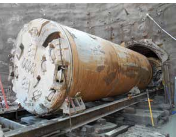
Figure 5: MTBM pushed through valve chamber portal
