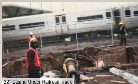
32" Casing Under Railroad Track
