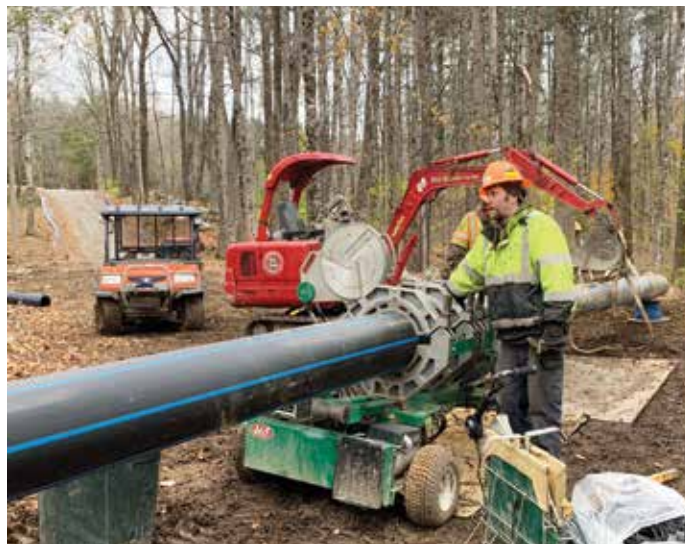
Fusing HDPE pipe string on site
