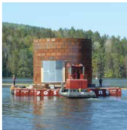
Figure 6: Water leg cofferdam structure with fiberglass soft eye
