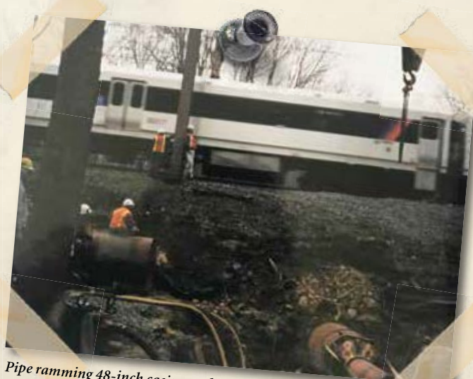
When directional drill is immobilized percussive power frees 2500 feet of 24-inch pipe with air hammer attached
