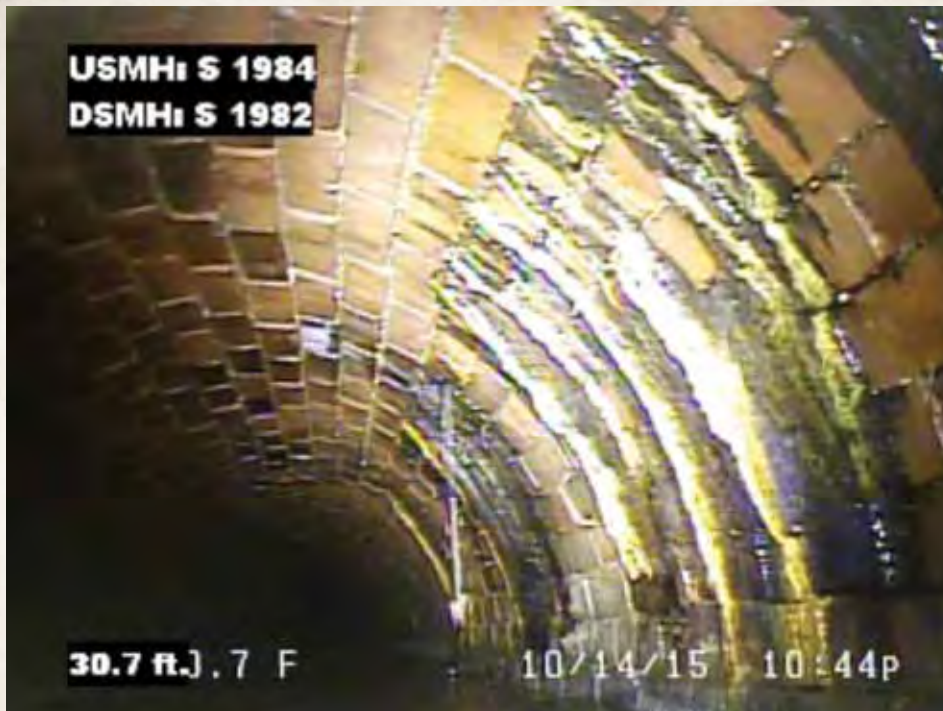
Figure 5. Active Infiltration and Mineral Deposits
