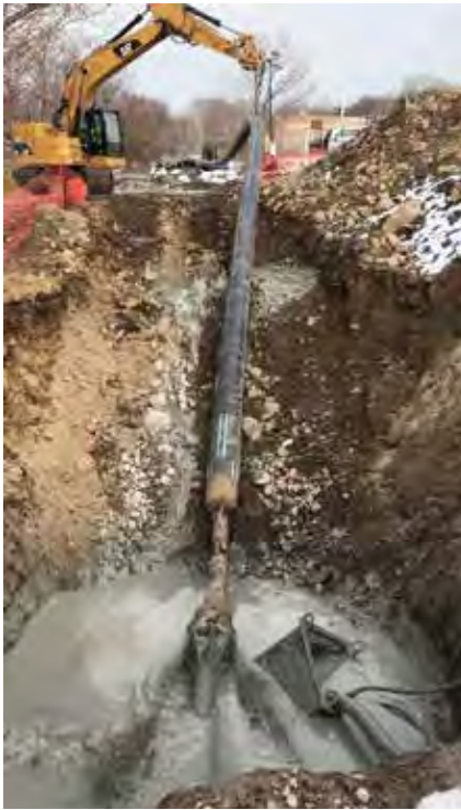
Figure 13: View of the east side work area at the beginning of pipe pullback
