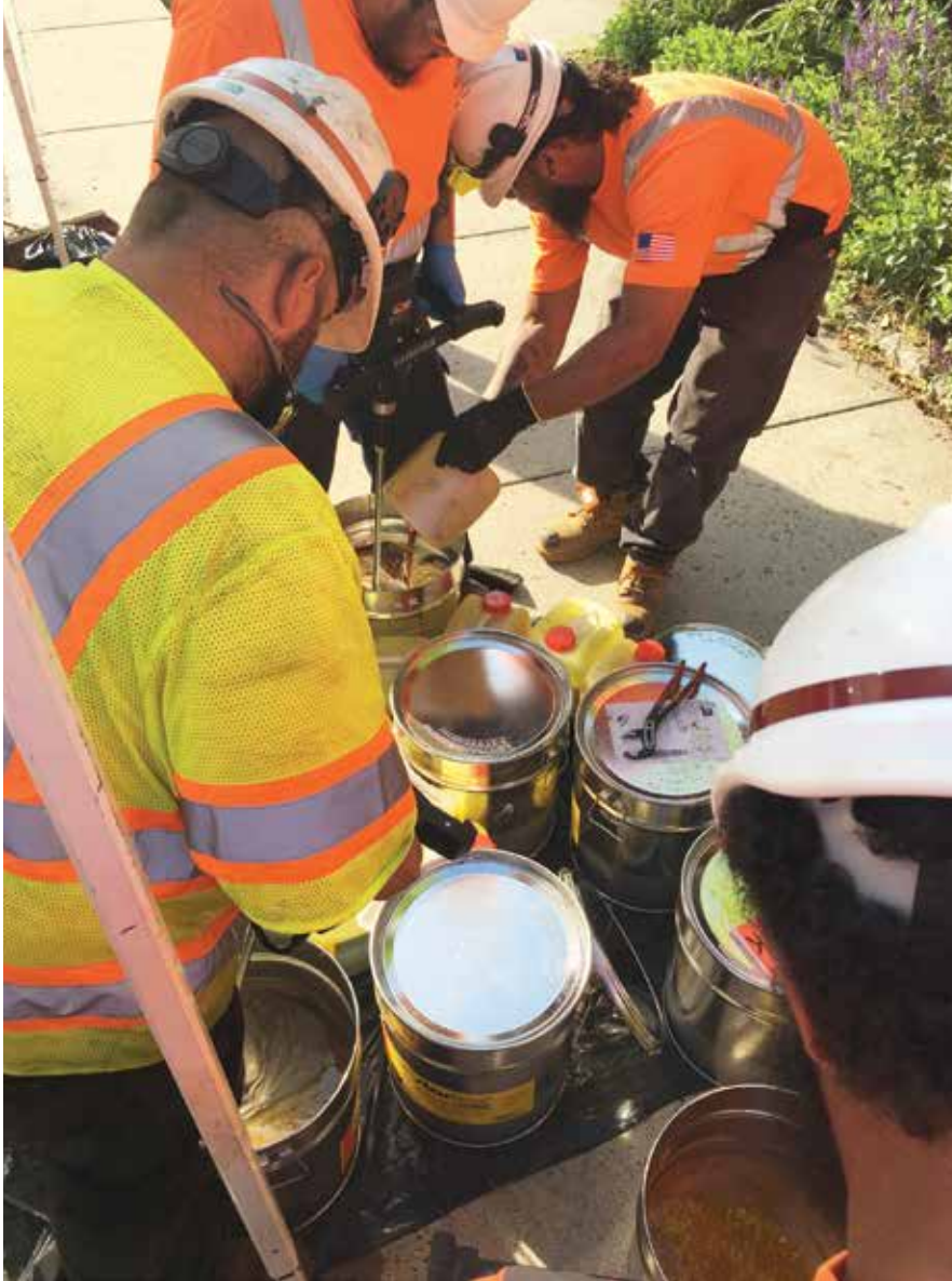
Mixing the Adhesive - The Clock Starts
