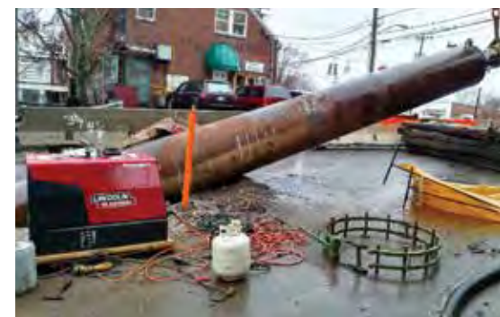
Figure 8: Installation of the conductor sleeve
