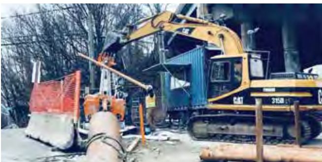
Figure 3: View of the HDD rig, overhead lines, I-95 bridge, site access and the conductor sleeve
