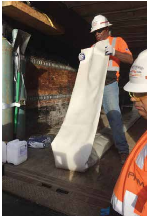
Preparing to Tape the End of Adhesive Filled Liner for Wet-Out
