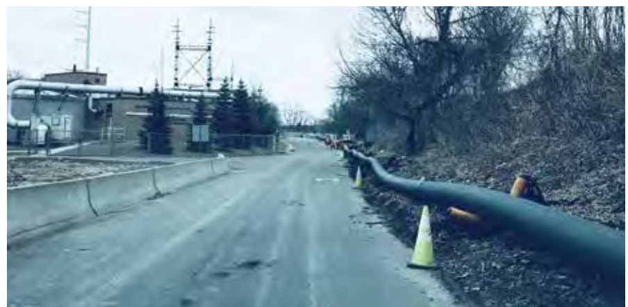
Figure 12: HDPE product pipe fused laid for pullback along Elaine road. WWPCF and I-95 are to the left and right side of the photograph respectively
