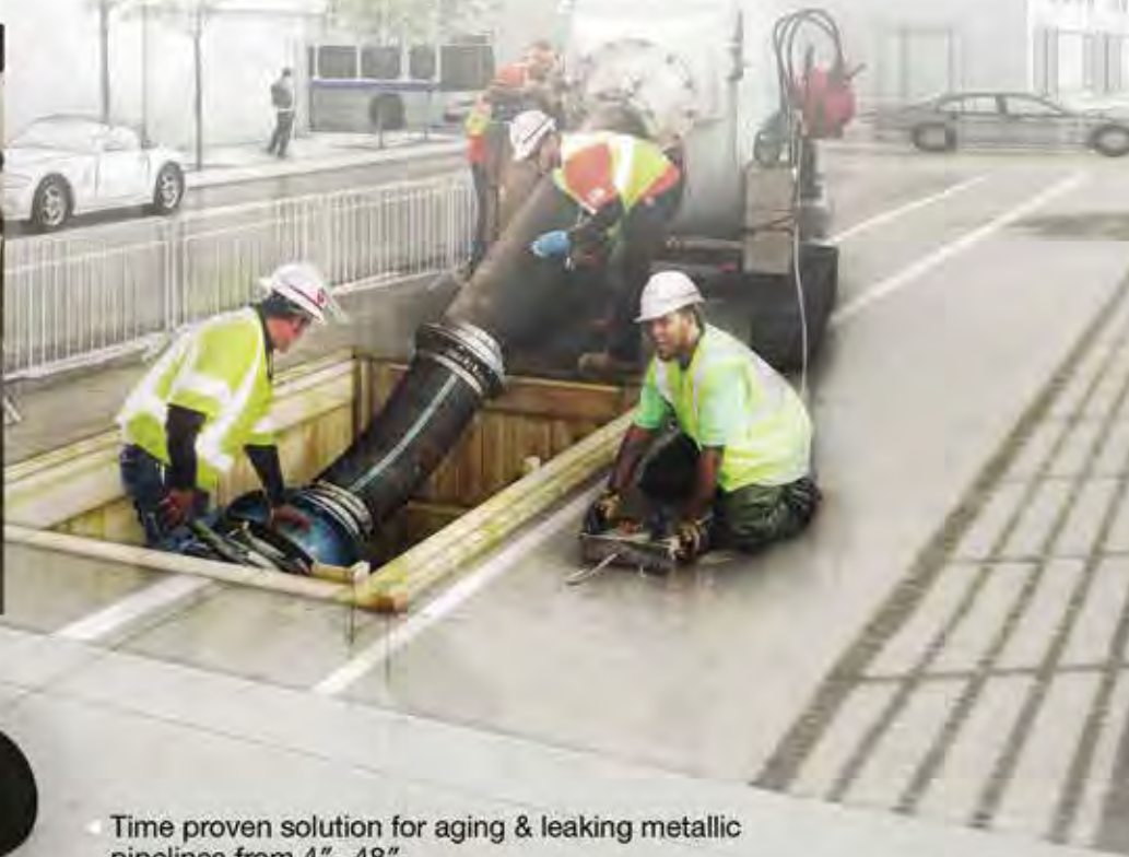
PPM / Starline holds the world record for the largest gas main ever lined. 36" Cast Iron Main, Seton Hall, NJ, November 2017
