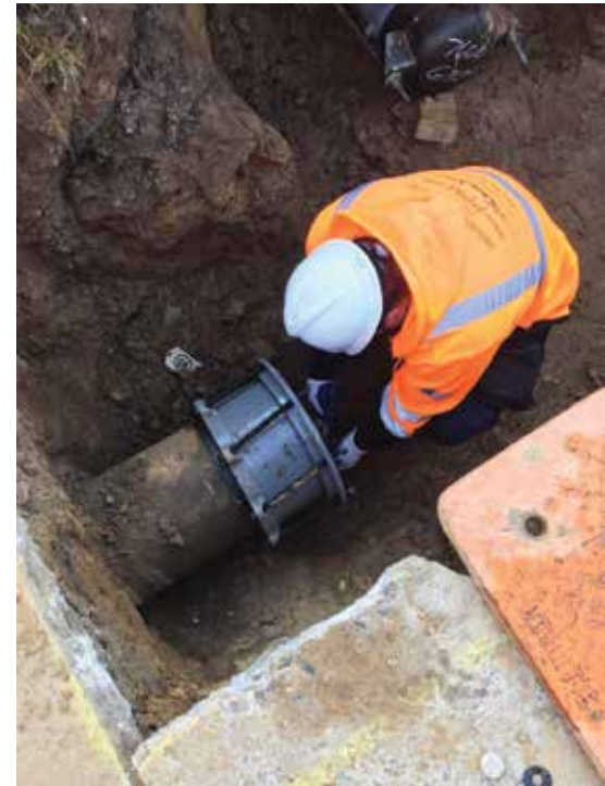
Removing the End Cap on the 12-inch Cast Iron Pipe
