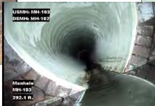
The egg-shaped sewer UVGRP liner was installed in seven sections completed in under two weeks
