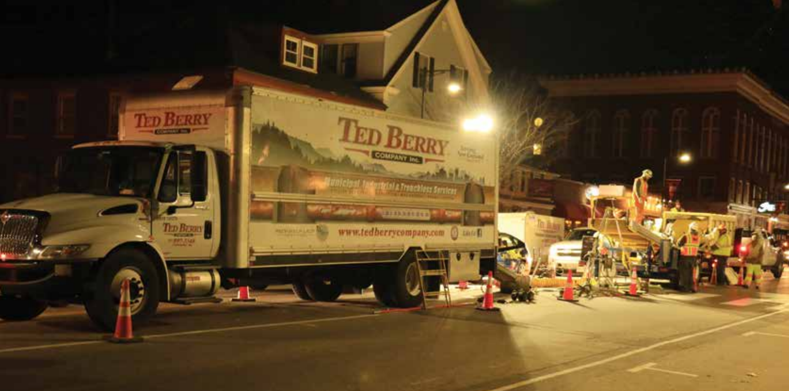
Each segment could be installed without bypass pumping if the work was done at night
