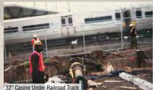
32" Casing Under Railroad Track
