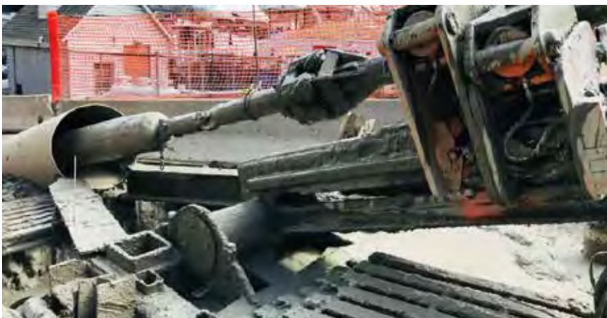
Figure 14: Product pipe pullback complete
