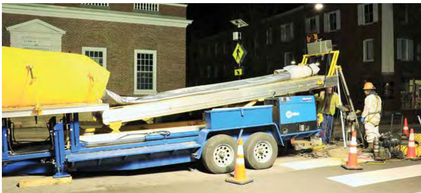
A motorized conveyor load system was used for liner placement into the existing manholes
