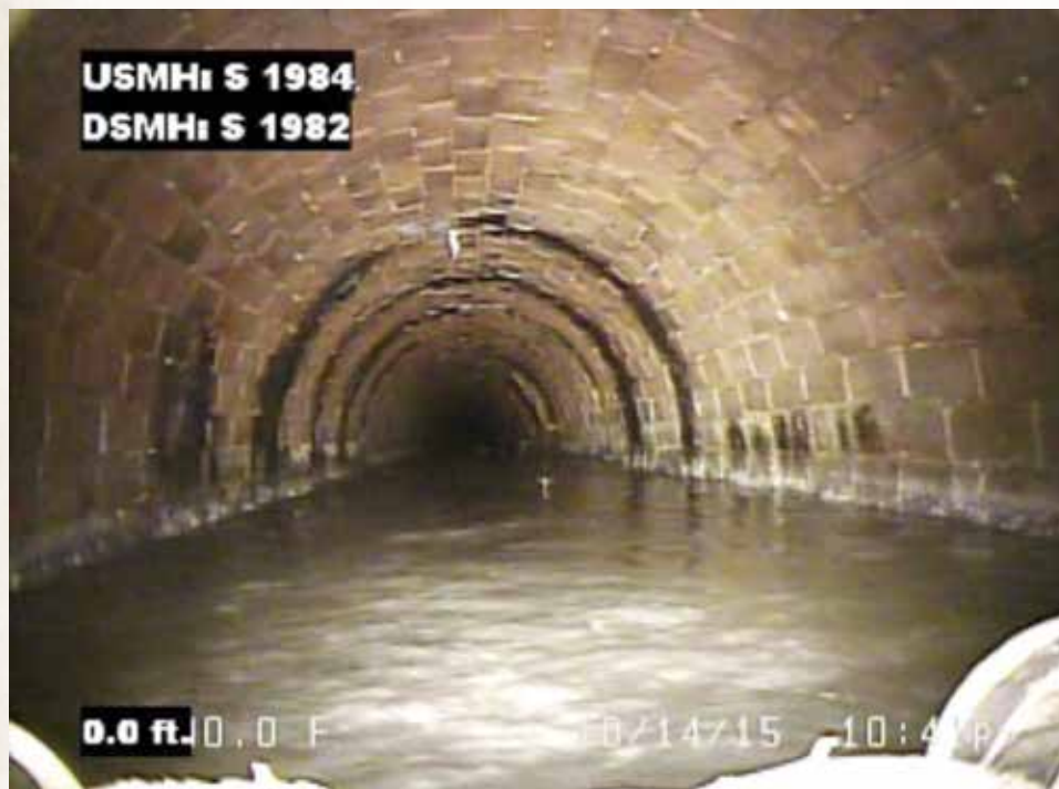
Figure 4. City of Revere Brick Trunk Sewer
