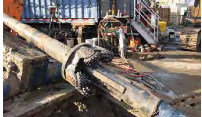
Figure 10: 22-inch diameter reamer on the HDD rig before starting the ream
