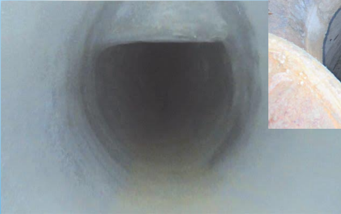
Liner application at Obstruction
