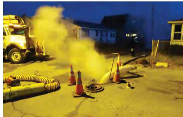
Lining & curing pipe into the night. The neighbors could not have been more hospitable
