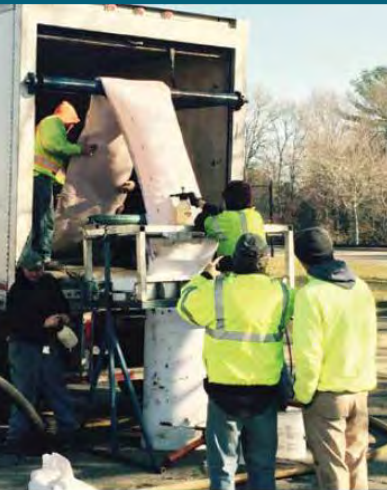
Lining & curing pipe into the night. The neighbors could not have been more hospitable
