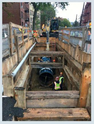
**Location:** South side of 31st Avenue between 35th Street and 36th Street **Operation:** Test Run using 20.0 L.F. test pipe with runners.
