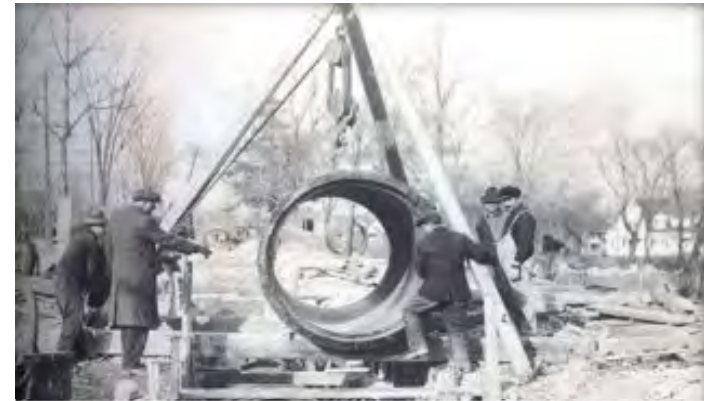
Original Pipe Installation
