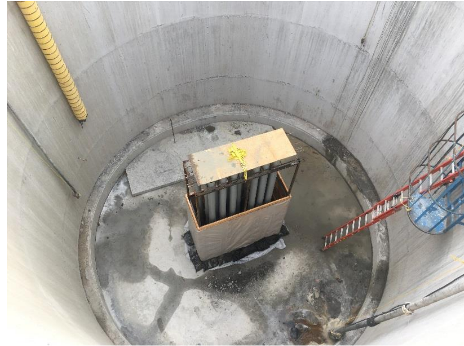
Box out for thermal grout around conduits and flowable fill for the rest of the shaft
