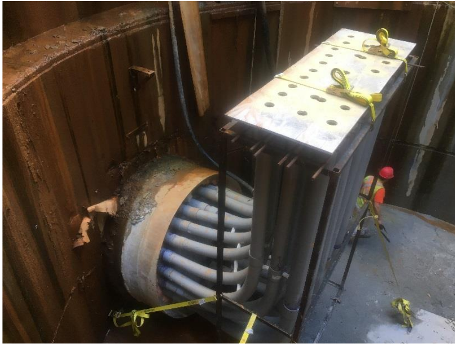
Conduit transition from tunnel to shaft
