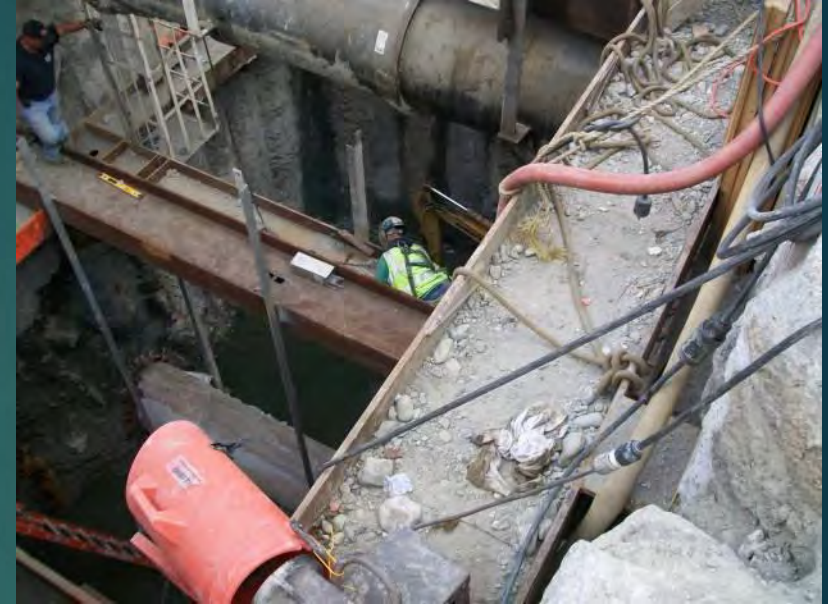
Utilities Supported in Place
