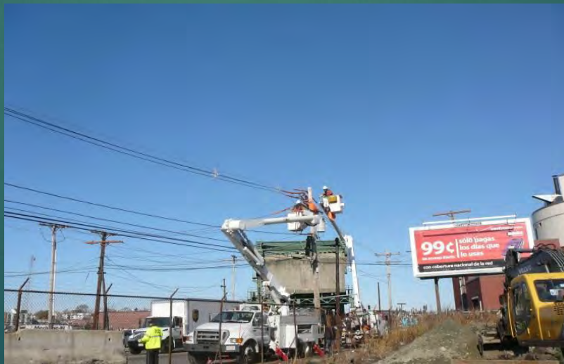
Overhead Wire Relocation
