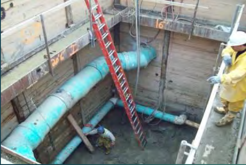
Sewer and Drain Relocation
