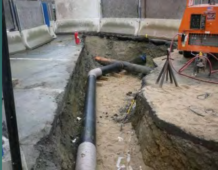
Gas Line Relocation
