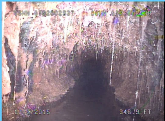
Pipe prior to cleaning with roots
