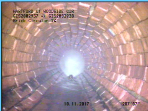
Pipe after cleaning and root removal
